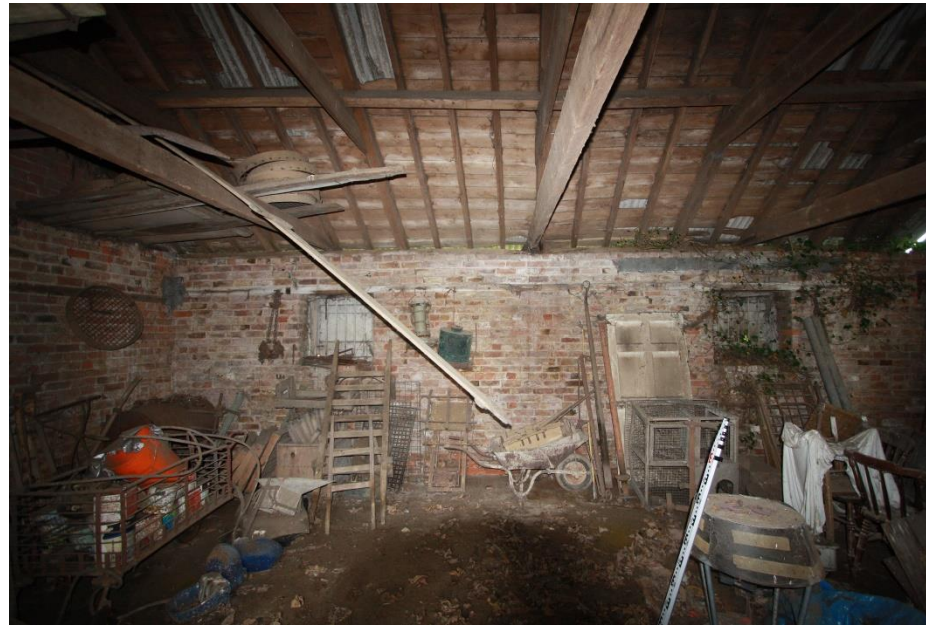
Image illustrating the good condition of the traditional roof to the brick built element of the barn
