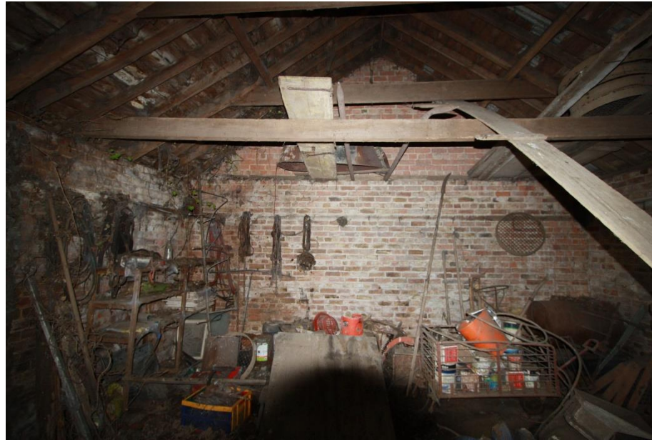
Image illustrating the good condition of the facing brickwork internally
