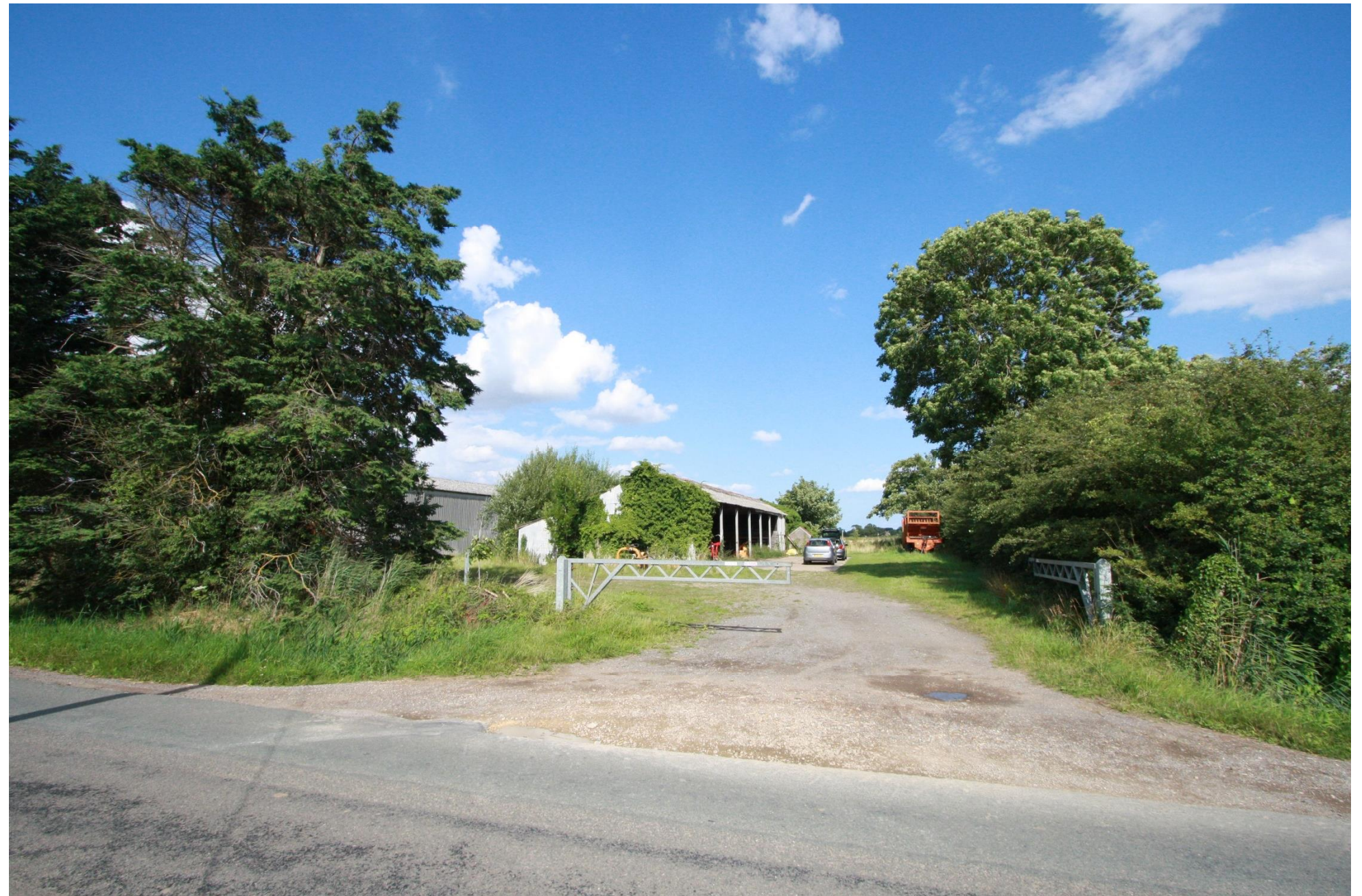
Existing Hedge to the South and Trees Along Money Bridge Lane
