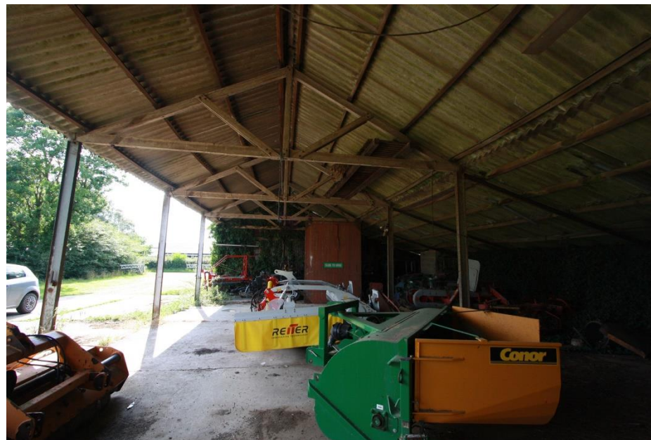
Image illustrating roof trusses with timber purlins and corrugated sheet roofing over
