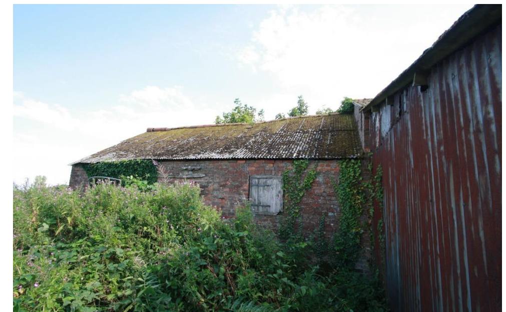
External image of brickwork northern elevation
