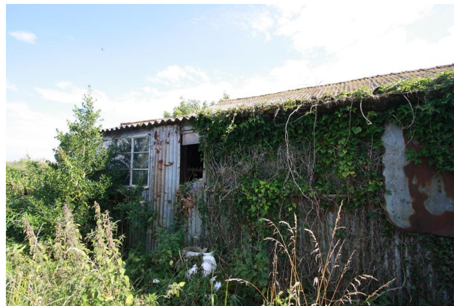
External image of steel windows and corrugated sheet metal
