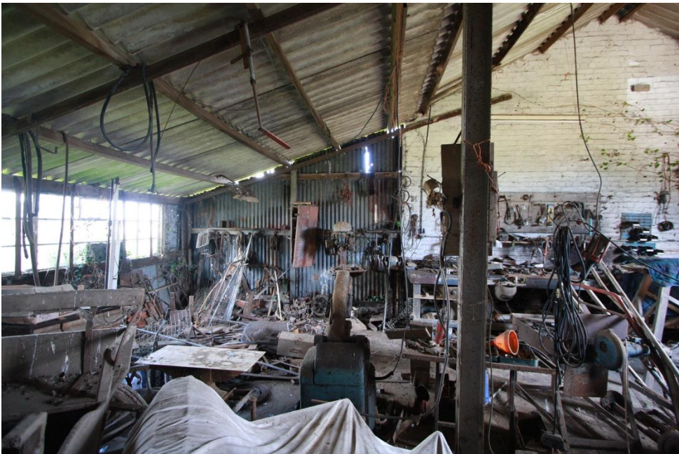
Image illustrating painted brick wall, corrugated metal wall and steel windows
