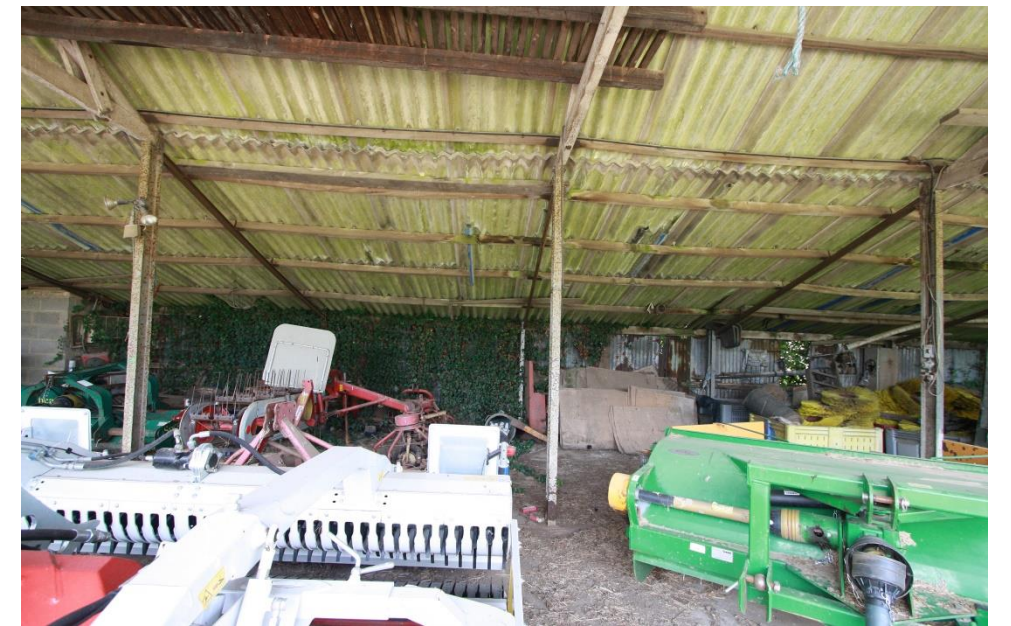
Image illustrating minor 'sag' to some timber purlins
