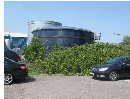
Effluent tanks seen from staff car park
