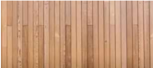
External- Timber Cladding
