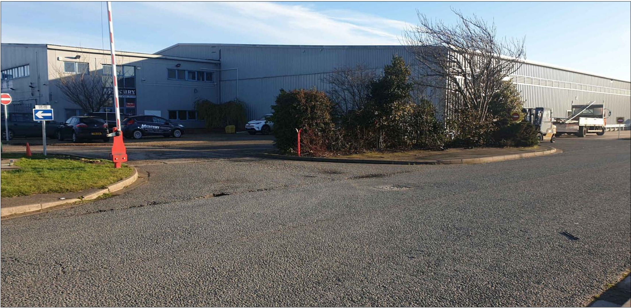
PHOTO 1 EXISTING CAR PARK ENTRANCE & EXIT
