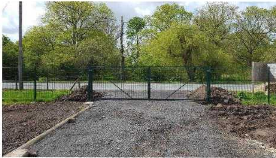
EXISTING SEASONAL CUSTOMER ACCESS VIA MAIN ROAD
