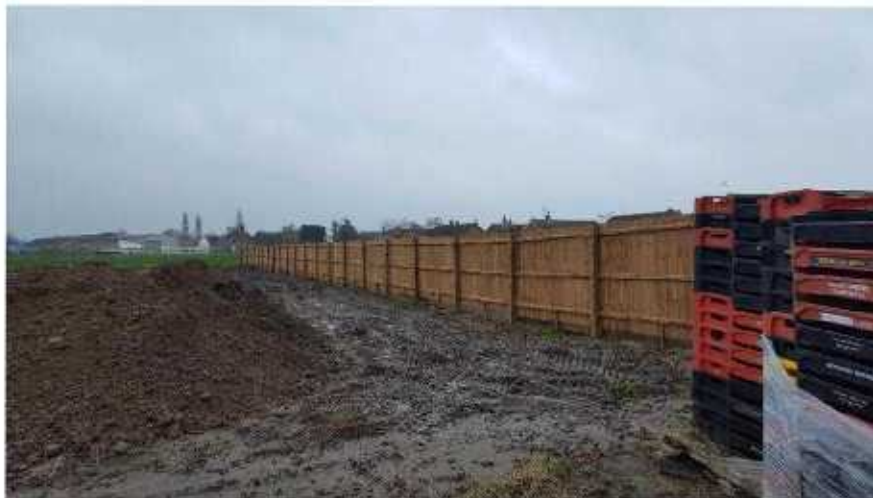
NEWLY ERECTED BOUNDARY FENCE TO SOUTH-EAST BOUNDARY
