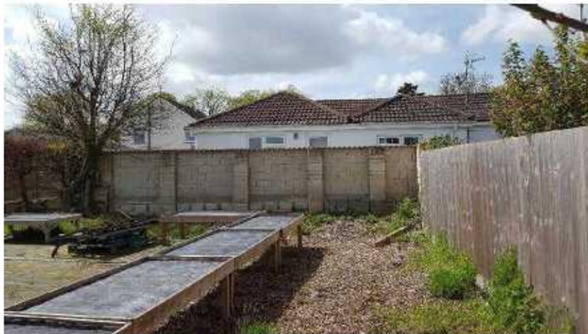
EXISTING BLOCKWORK BOUNDARY WALL REAR OF No.125 MAIN ROAD
