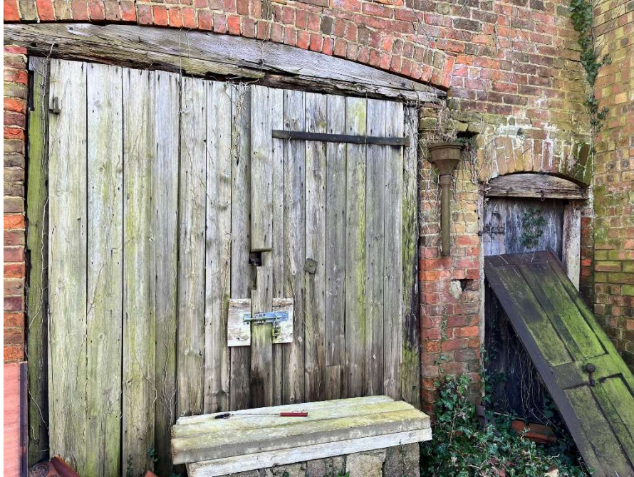
Main door on the southwest side, steel door from the smokery to the right of the picture
