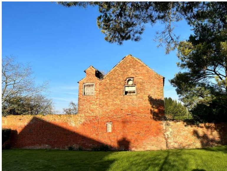
View from the southeast, smokehouse to the left
