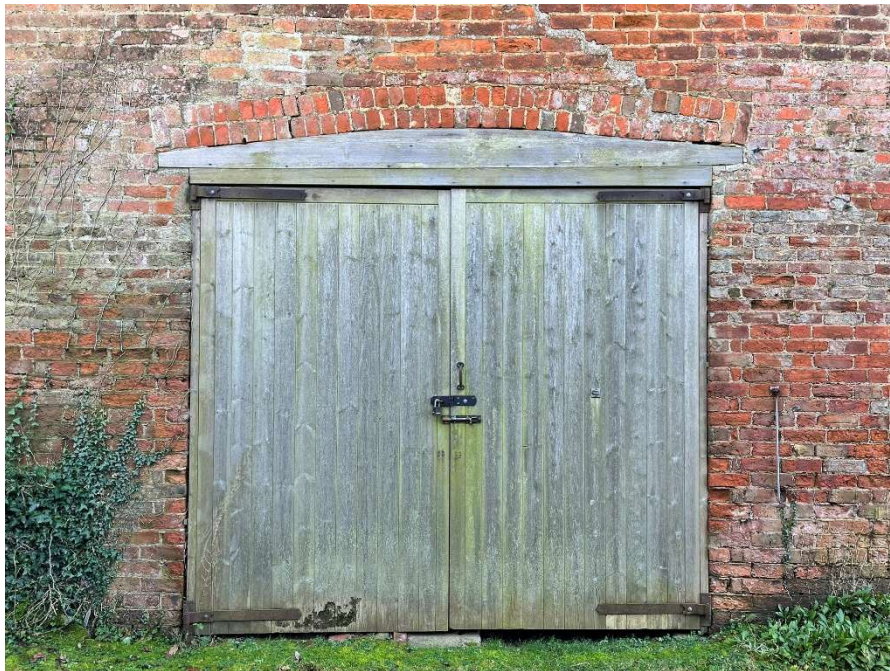
Door to the northeast side of the barn, facing the road
