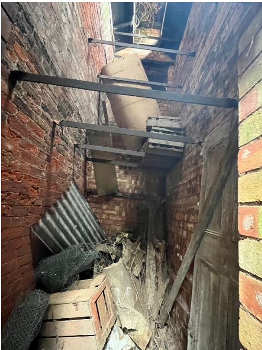
Plate One: Internal arrangement of bars for suspension of items with good air flow.
