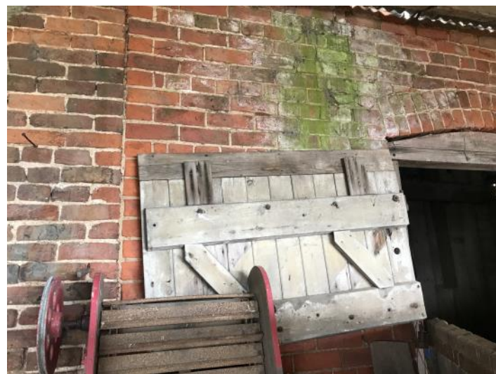
Fig. 8 : Photo of Barn 2 (south elevation) showing original full height opening
