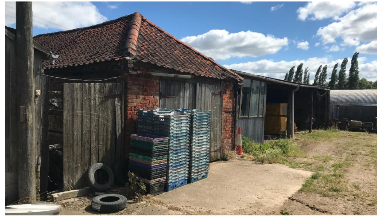
Fig. 4 Photograph showing the single storey barn and adjacent lean-to storage (view of south elevation)
