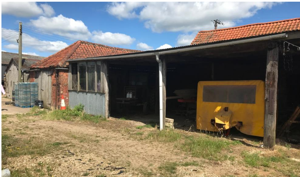
Fig. 5 Photograph showing lean-to storage adjacent to both barns (view of the south elevation).
