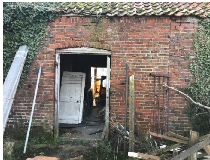
Fig 9. Photo of Barn 2 (north elevation) Showing original full height opening
