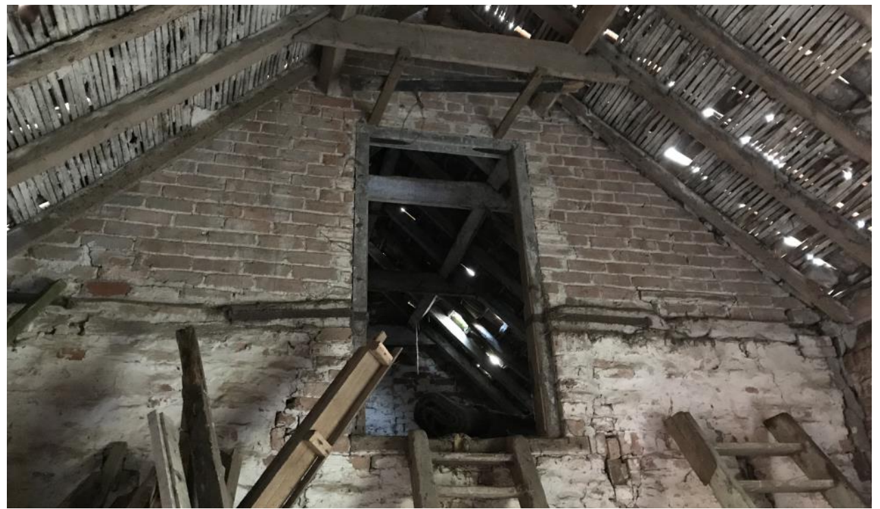
Fig. 6 Photograph showing the internal view of the first floor in the 2 storey barn.
