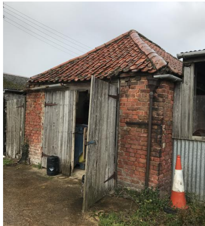
Fig. 11 : Photo's of Barn 1 (south elevation) Showing existing brickwork and roof tiles
