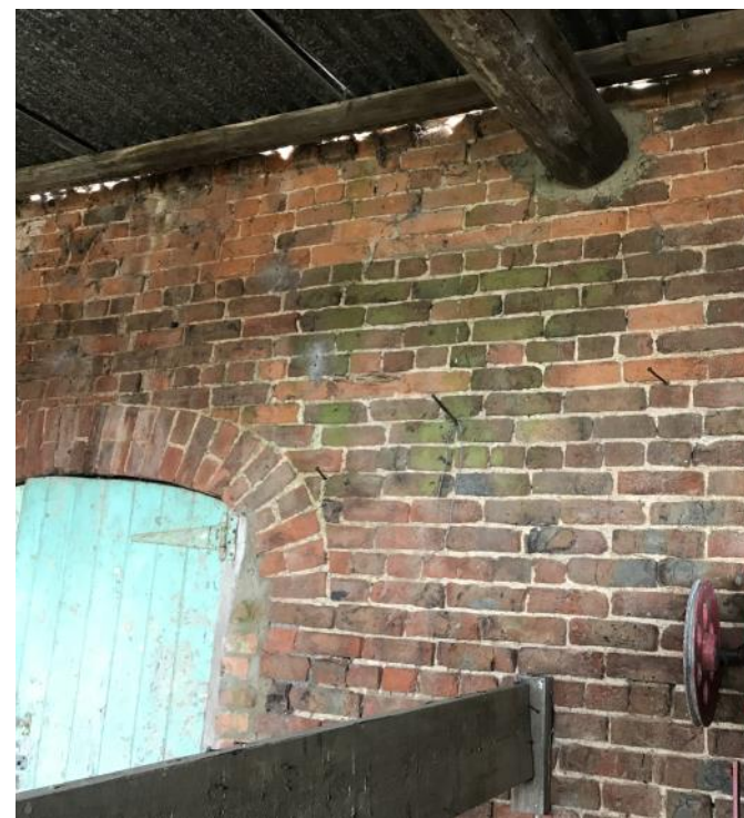
Fig 12. Photo of Barn 2 (south elevation) showing existing brickwork
