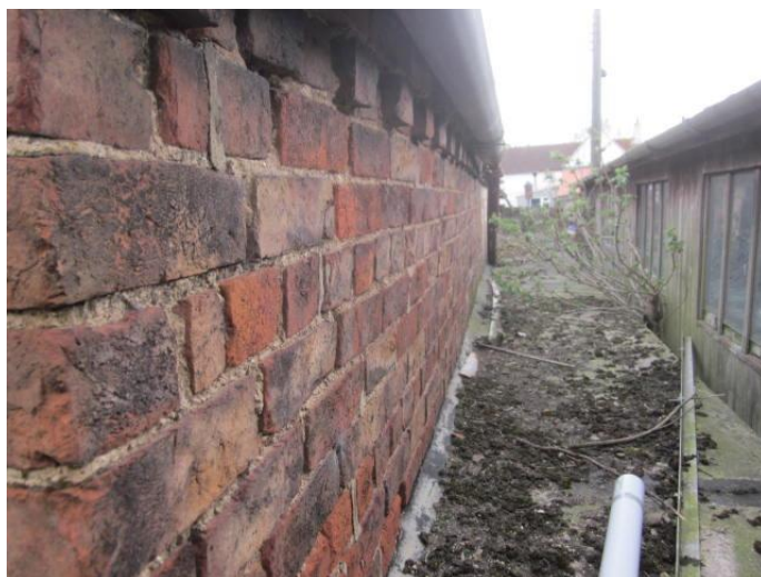
Photograph # 5 (Barn 1 – West Facing Elevation) – Dryer Tunnel Structure visible
