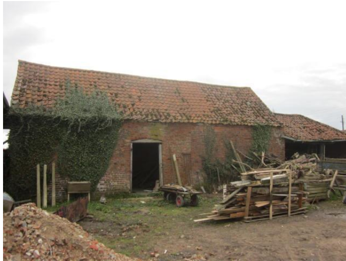
Photograph # 10 (Barn 2 – North Facing Rear Elevation)
