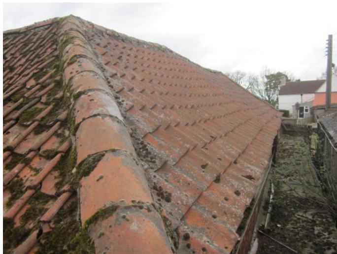
Photograph # 9 (Barn 1 – Roof - External)
