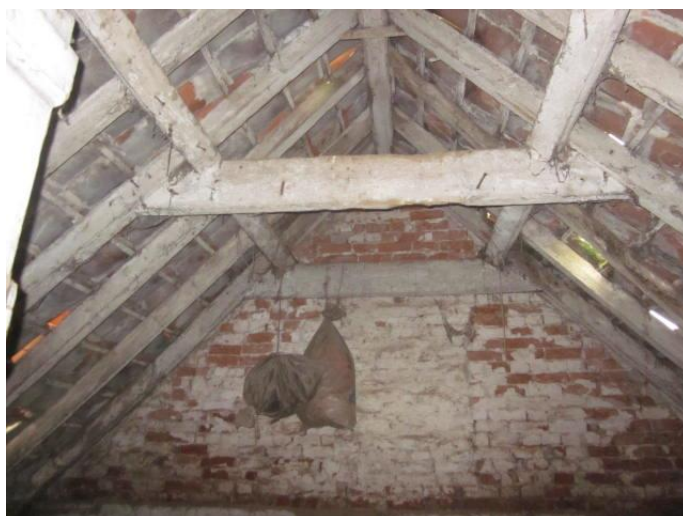
Photograph # 18 – (Barn 2 – Roof - Internal)
