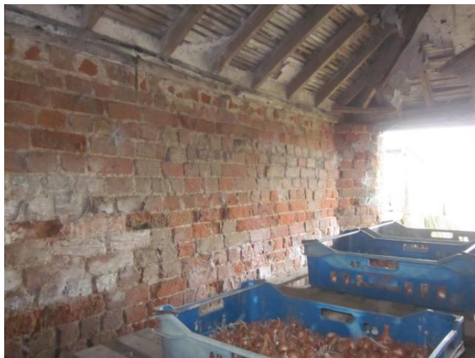
Photograph # 4 (Barn 1 – West Facing Elevation)
