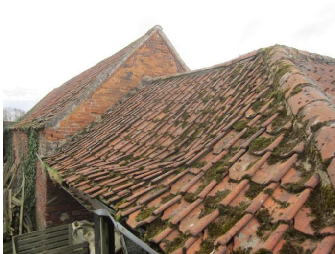
Photograph # 8 (Barn 1 – Roof - External)
