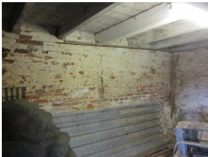
Photograph # 21 – (Barn 2 – First Floor (underside))
