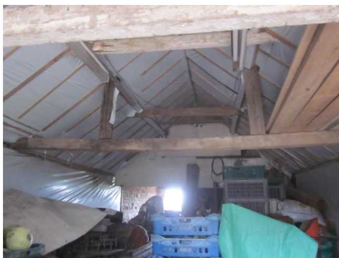
Photograph # 6 (Barn 1 – Roof - Internal)
