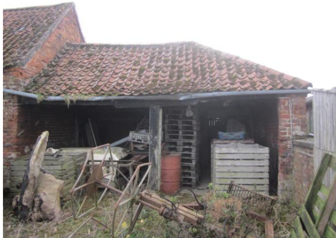
Photograph # 2 (Barn 1 – North Facing Rear Elevation)
