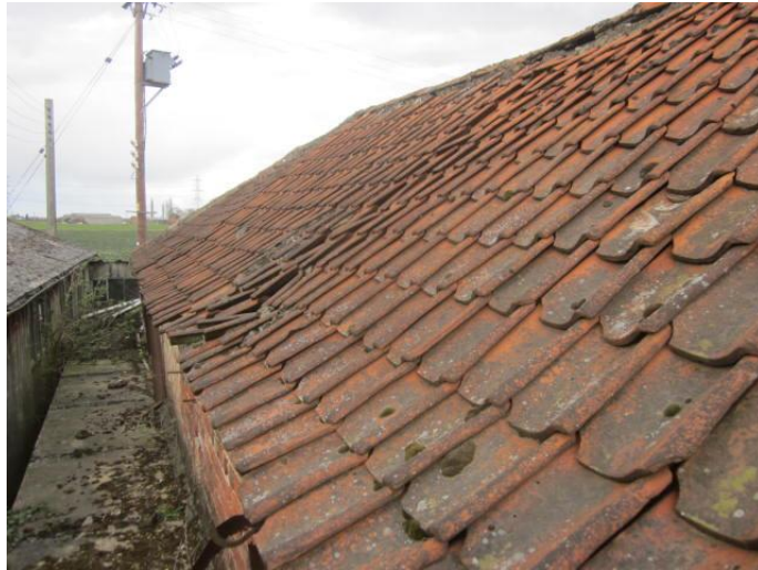
Photograph # 7 (Barn 1 – Roof - External)
