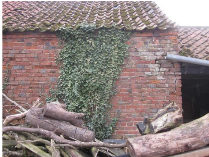
Photograph # 13 (Barn 2 – North Facing Rear Elevation)
