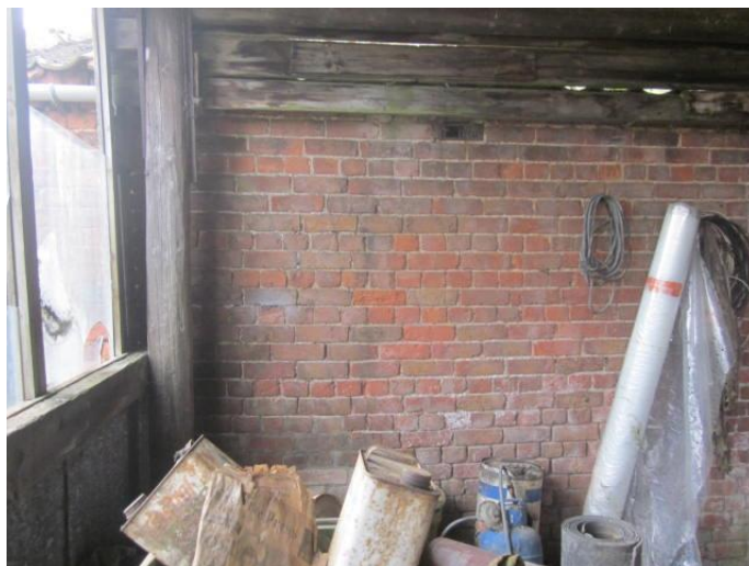
Photograph # 3 (Barn 1 – East Facing Elevation)
