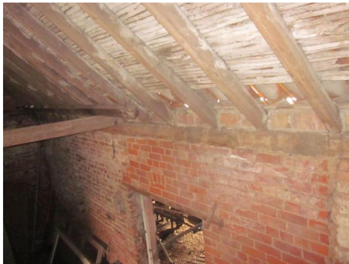
Photograph # 20 – (Barn 2 – Roof - Internal)
