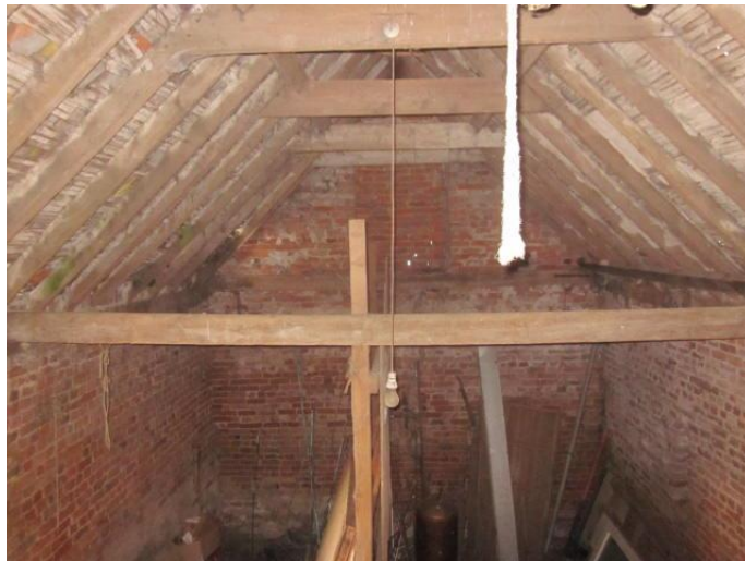
Photograph # 19 – (Barn 2 – Roof - Internal)
