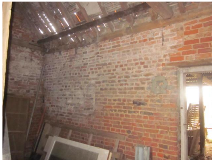
Photograph # 14 (Barn 2 – South Facing Front Elevation - Internal)
