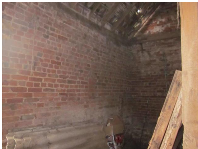
Photograph # 15 (Barn 2 – North Facing Rear Elevation - Internal)
