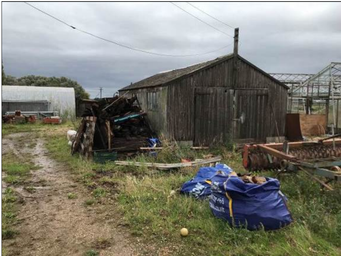
Fig 6 – view to east along south boundary with wooden shed with CBA roof beyond
