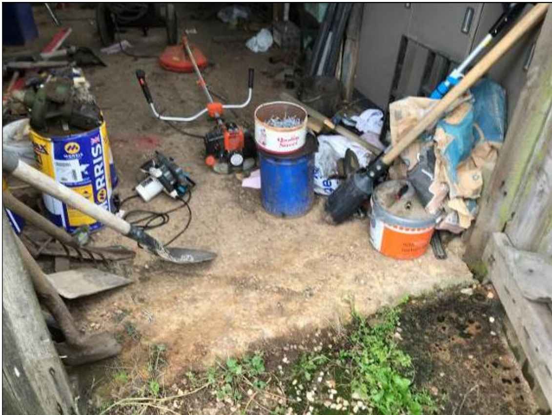
Fig 8 – concrete floor common in all sheds and barns
