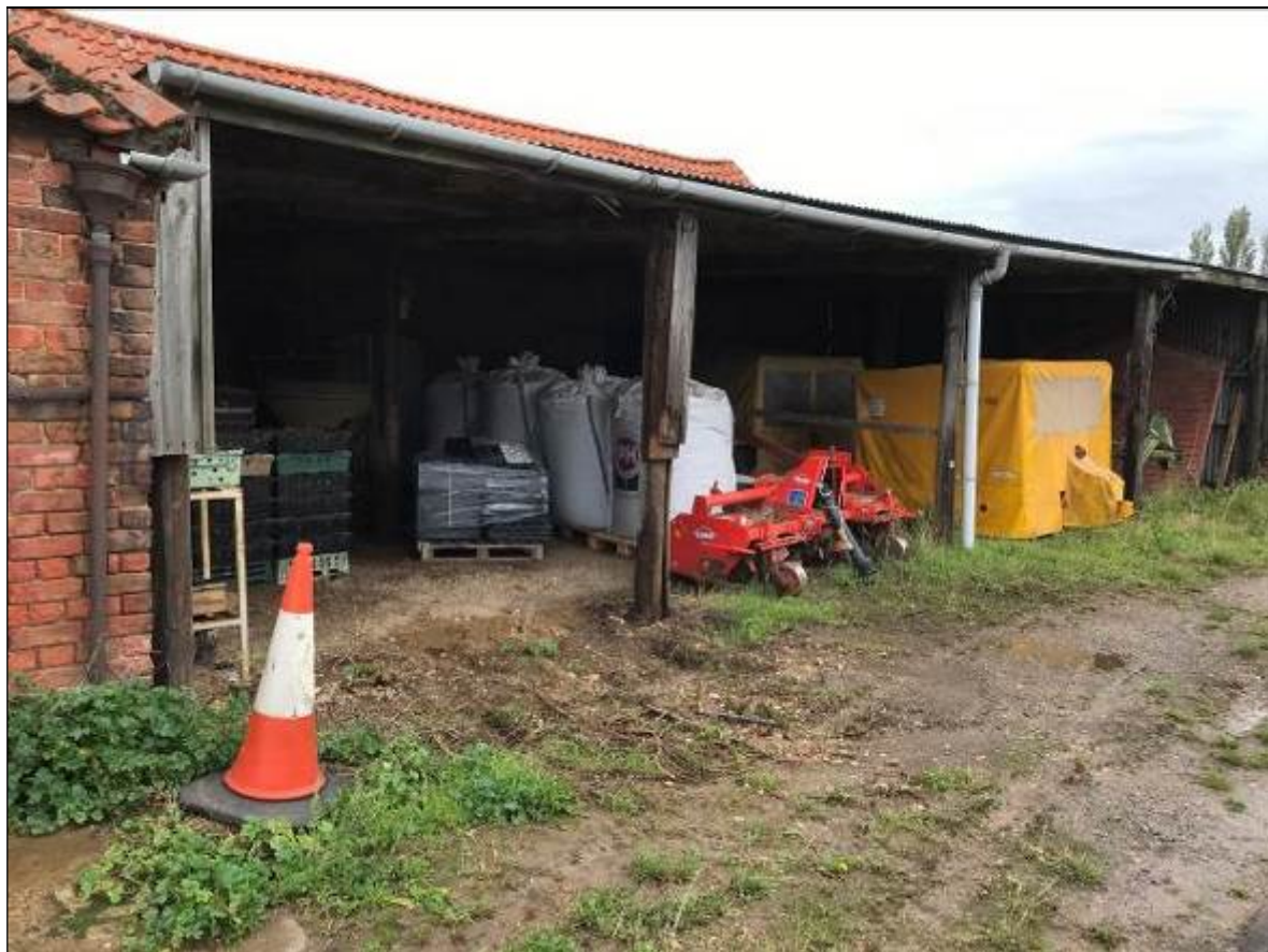
Fig 7 – view to north east of open-sided barn
