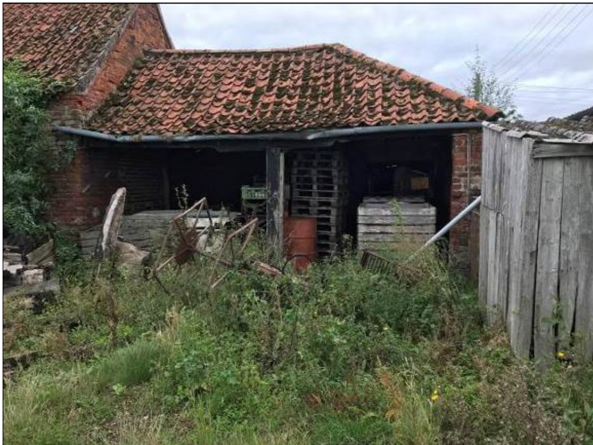
Fig 9 – view to south of north elevation
