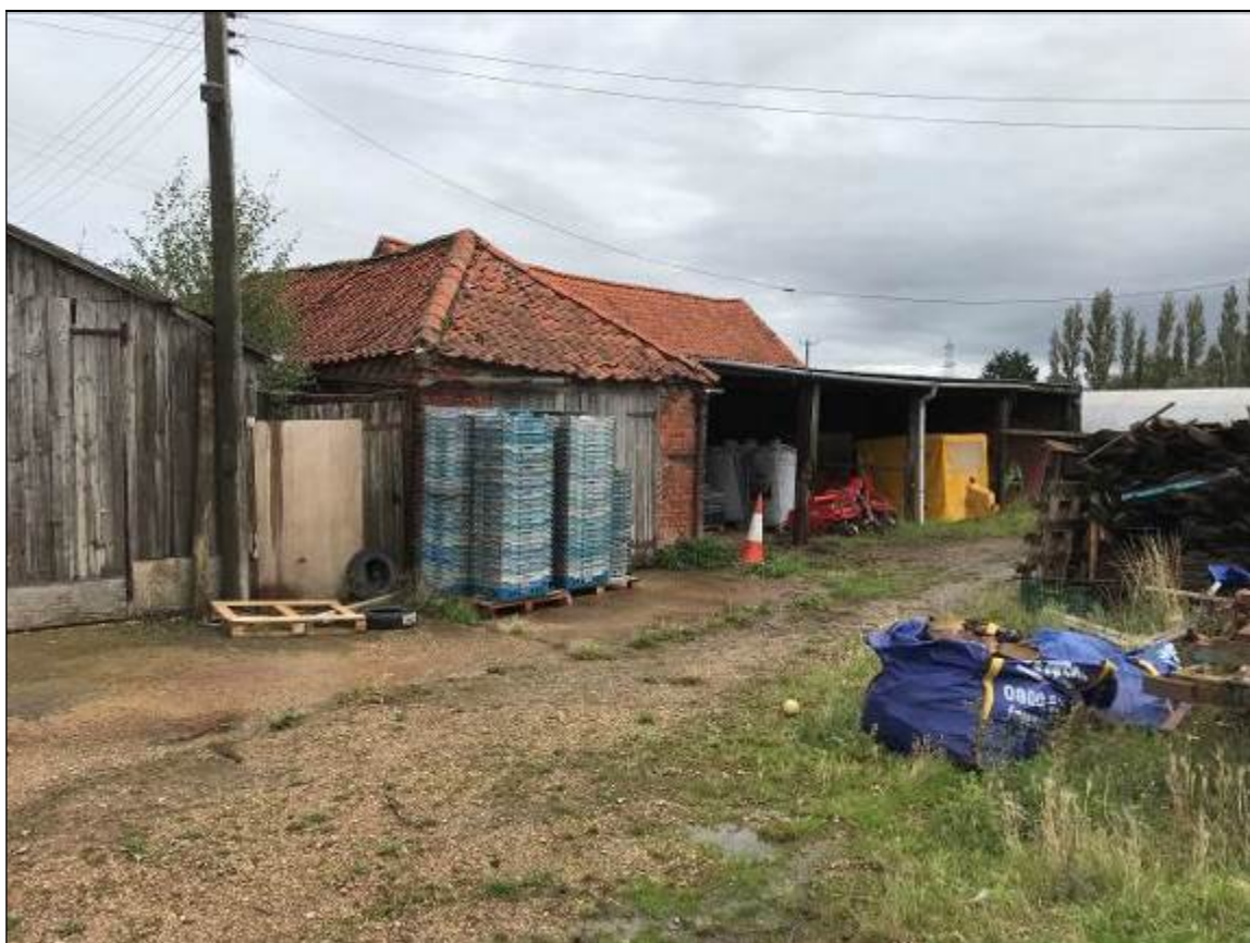
Fig 5 – view to northeast along south boundary
