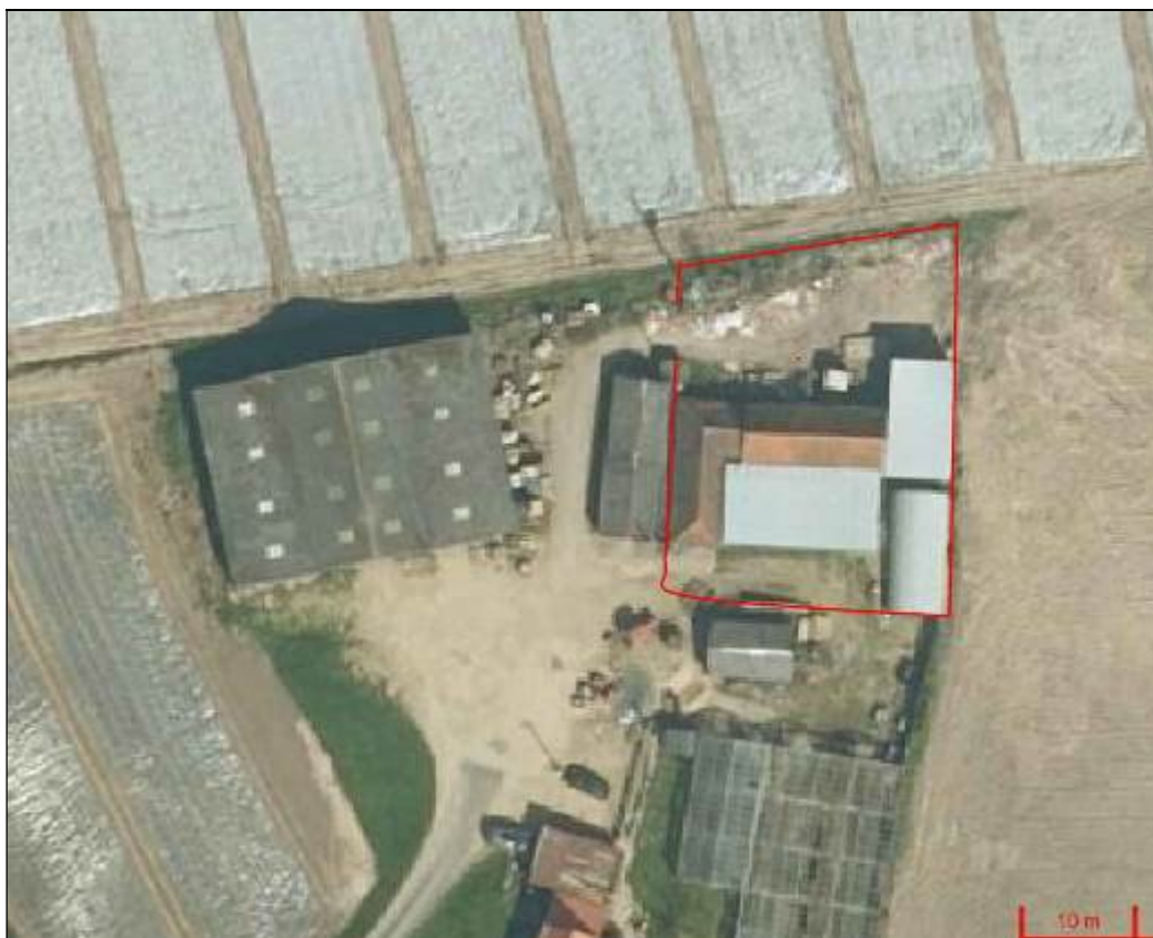
Fig 3 – aerial view of site
