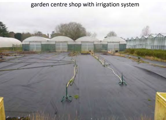
Photo 6 - Geotextile membrane covering display area outside garden centre shop with irrigation system
