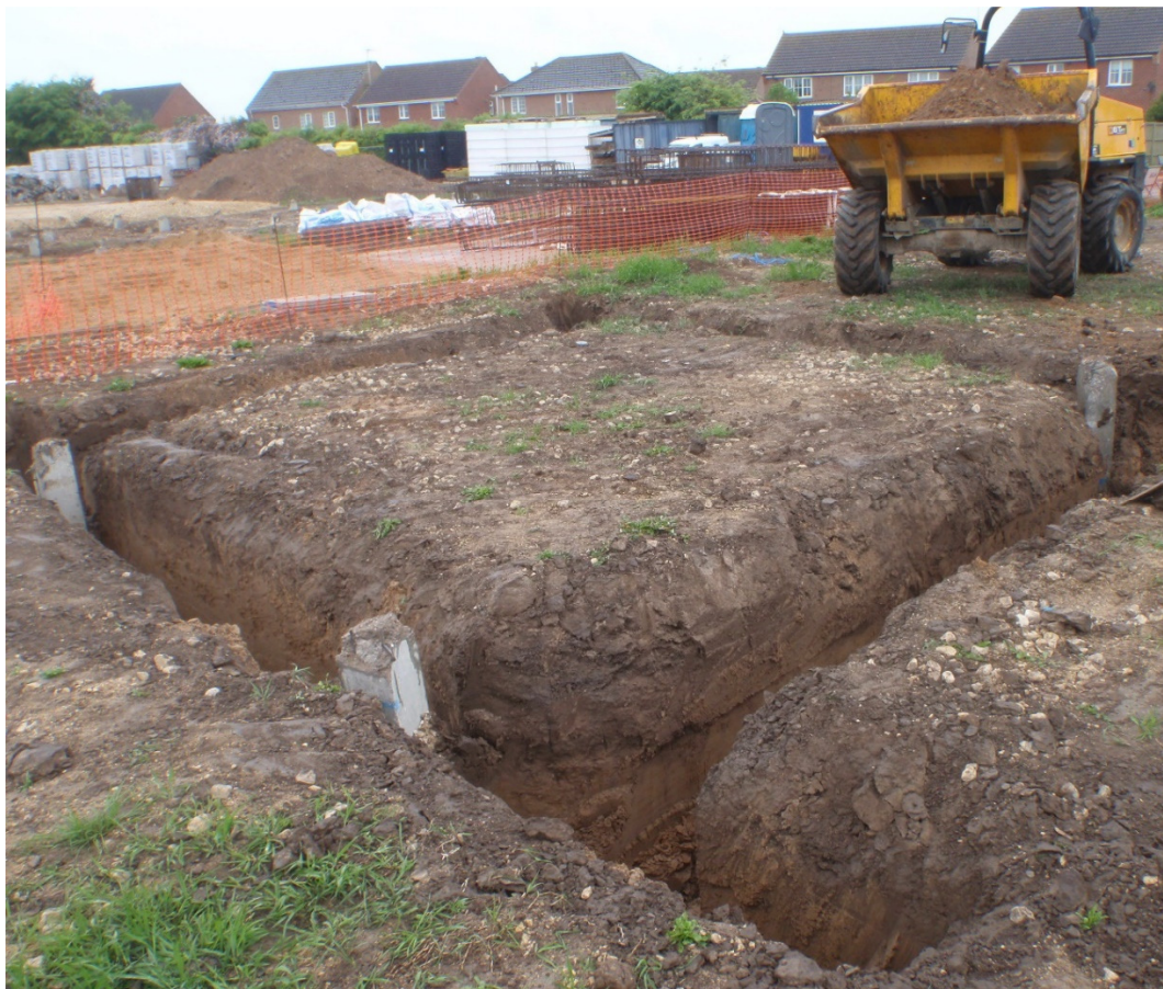
Plate 8 Plot 2 garage fully excavated, looking west
