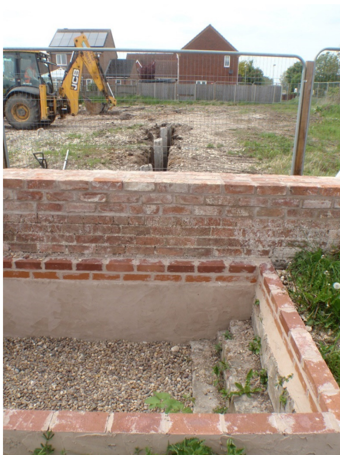
Plate 4 Looking west across the west wall of the pool to Plot 2
