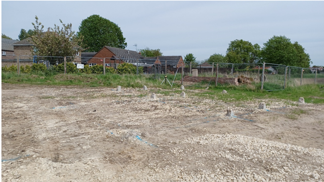
Plate 1 Pre excavation shot looking northeast across Plot 2 towards the burial ground (piles already in place)
