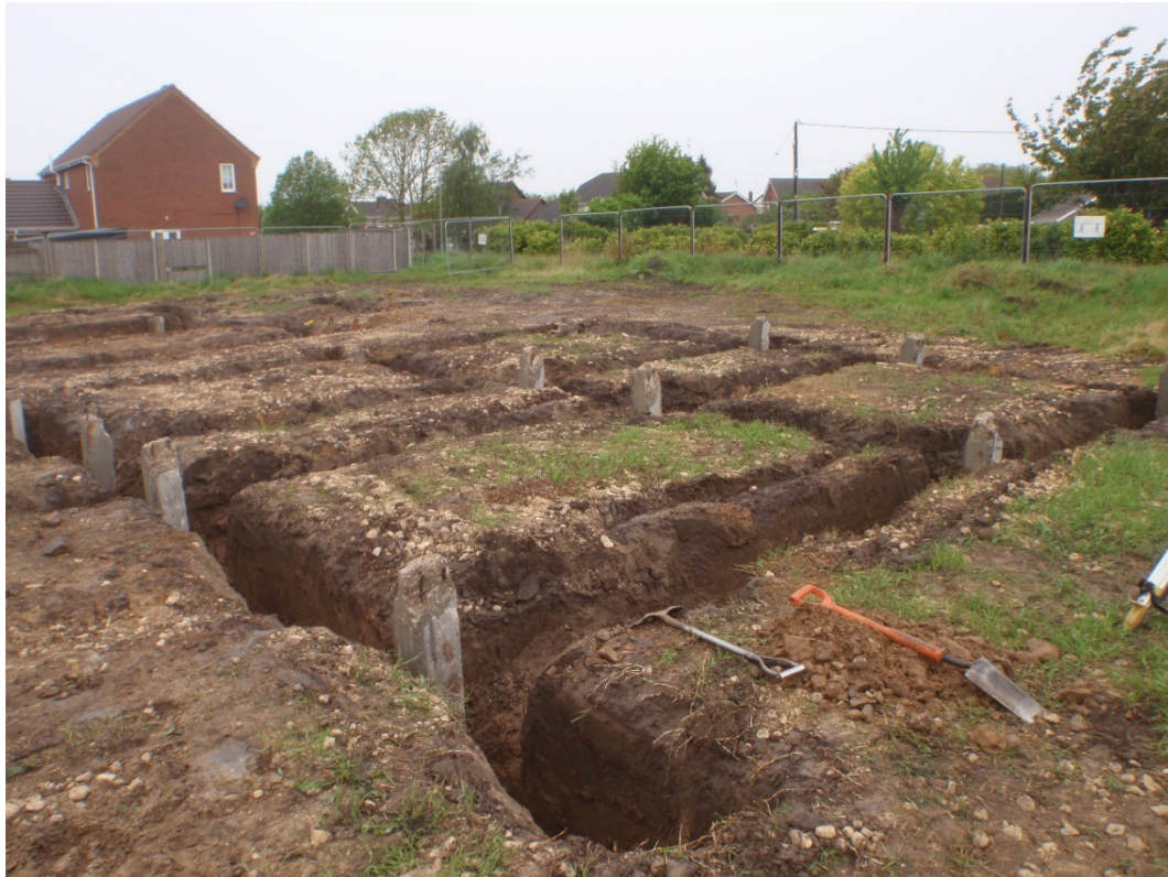
Plate 7 Plot 2 fully excavated, looking northwest
