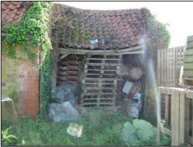
Fig 6: Building N° 3 north east aspect
