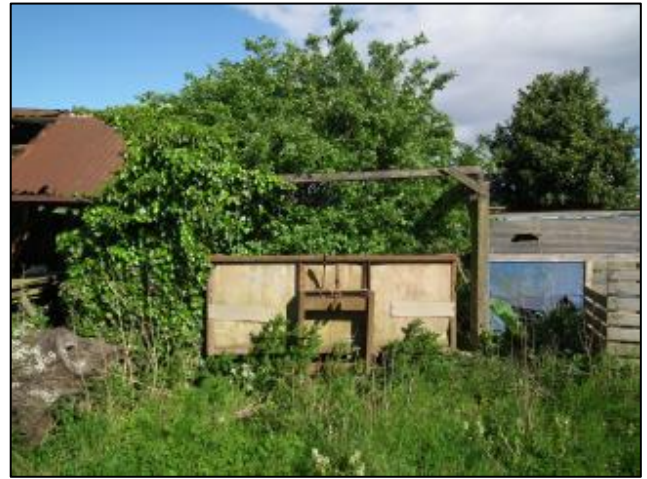
Fig 7: The main building from Water Gate
