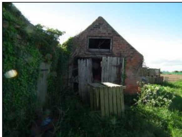
Fig 5: Building N°2 south east aspect
