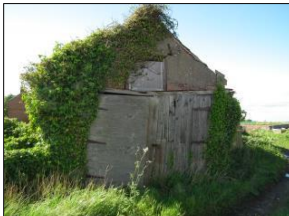
Fig 4: Building N°1 south east aspect
