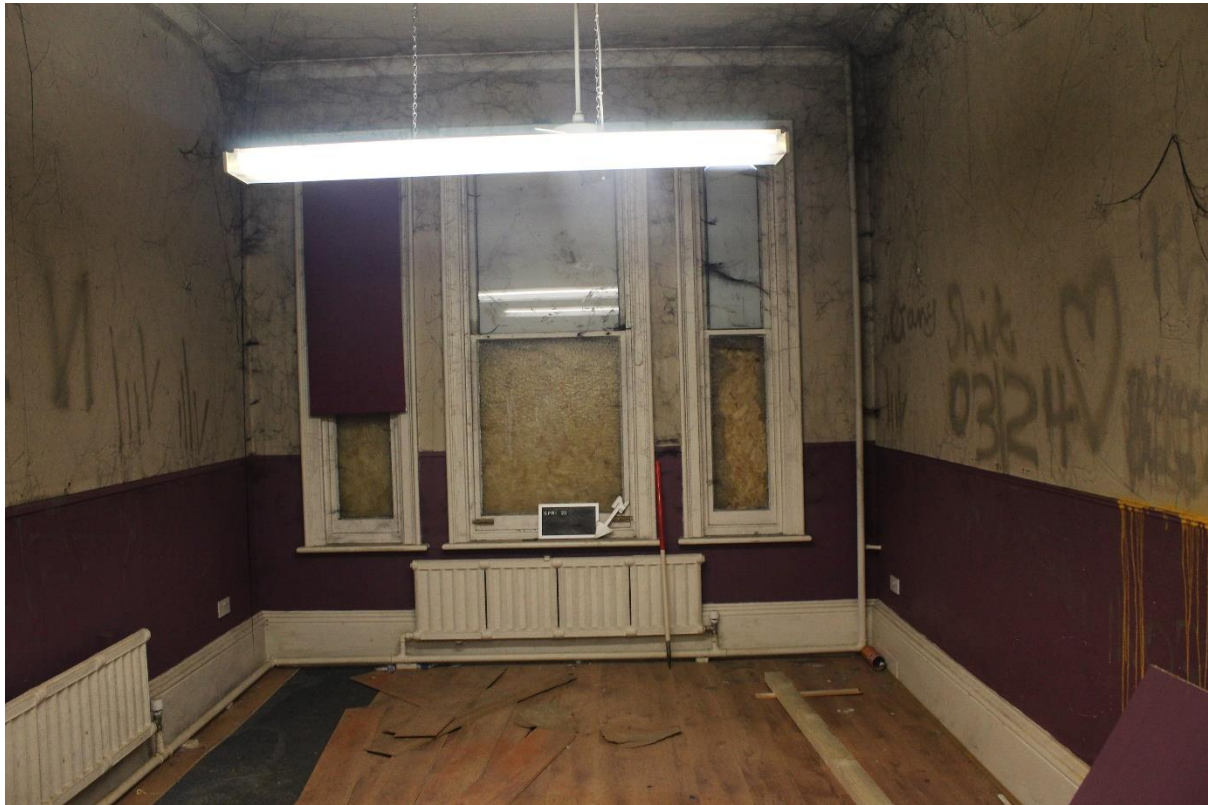
Plate 13: Gym looking southeast.
