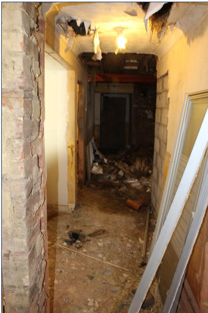
Plate 24: Hallway looking northwest.
