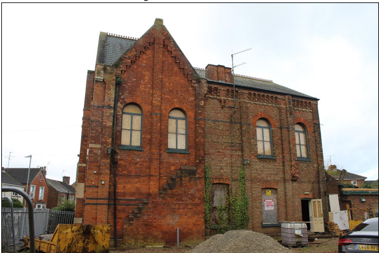
Plate 4: northeast elevation looking southwest.
