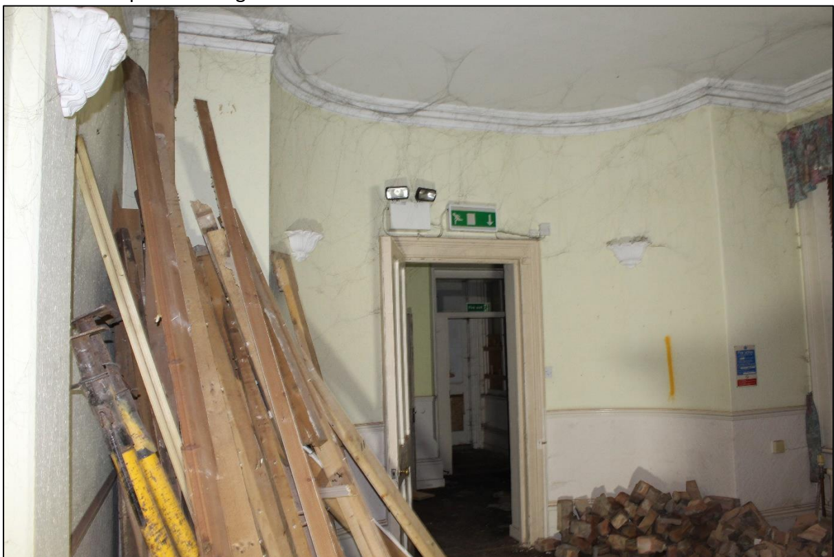
Plate 22: Reception looking southeast.
