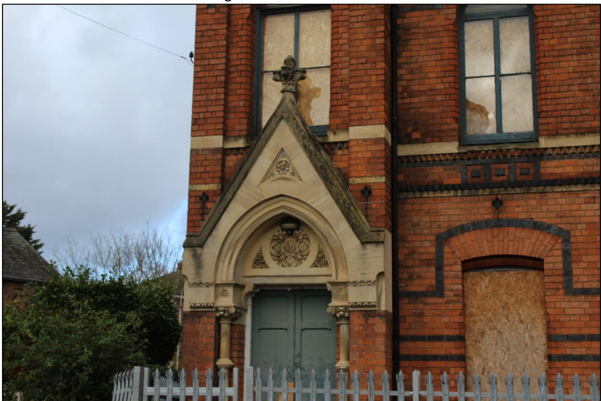
Plate 2: Southeast elevation, detail of entrance porch looking northwest.
