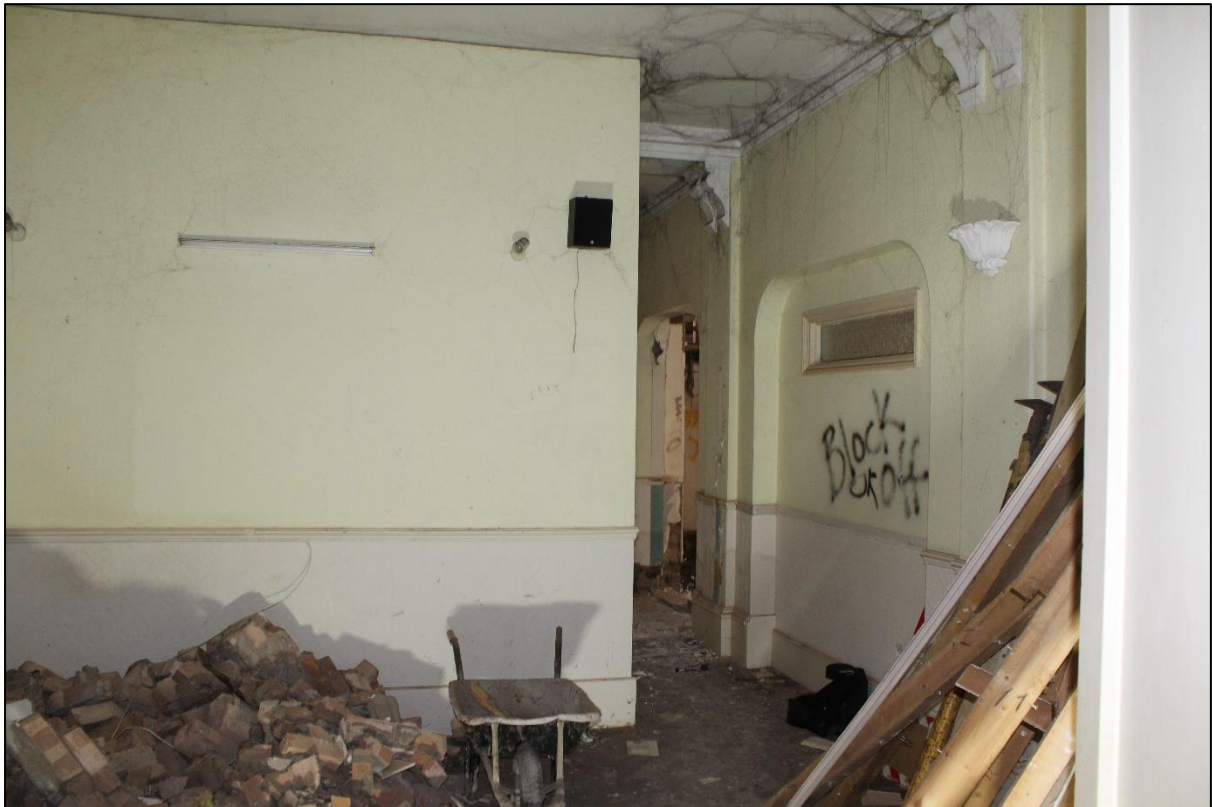
Plate 21: Reception looking north.
