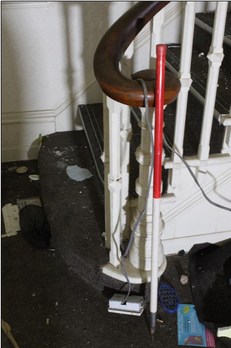
Plate 16: Stair balustrade detail within entrance hall.
