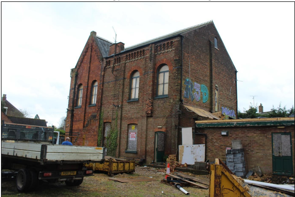
Plate 7: northeast elevation looking southwest.
