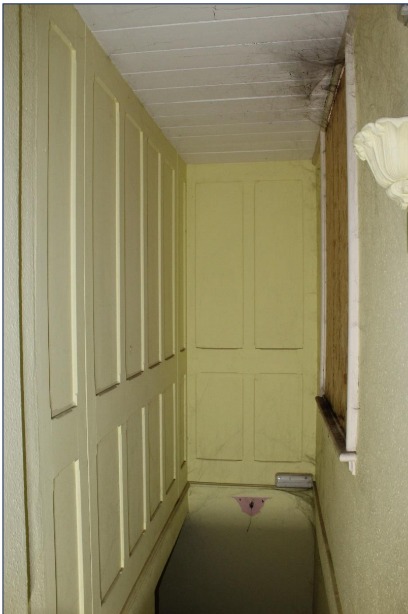
Plate 33: Stairwell to entrance hall looking northeast.
