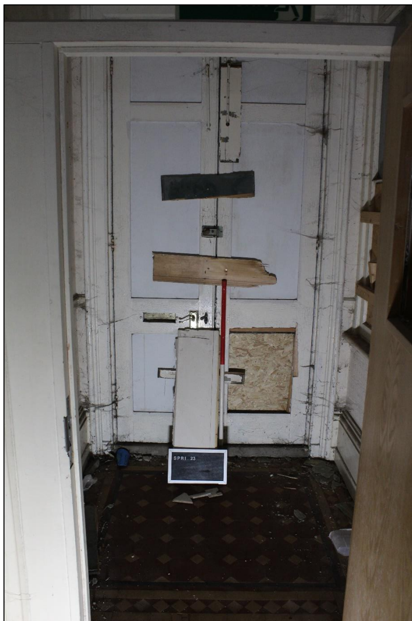
Plate 18: Lobby looking southeast.
