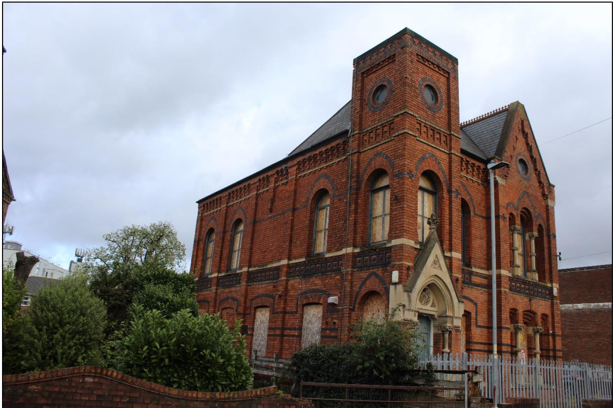
Plate 3: Southwest elevation looking north.
