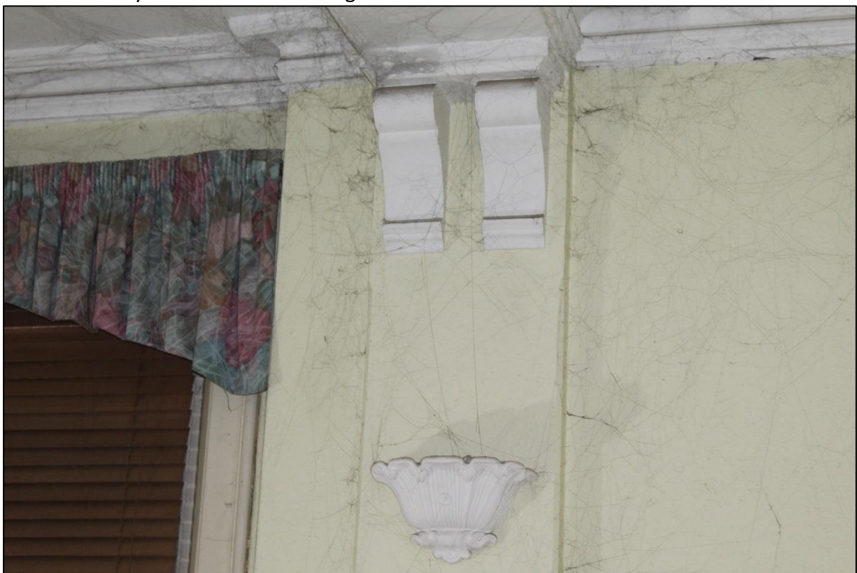
Plate 20: Corbel and coving detail reception, looking southwest.
