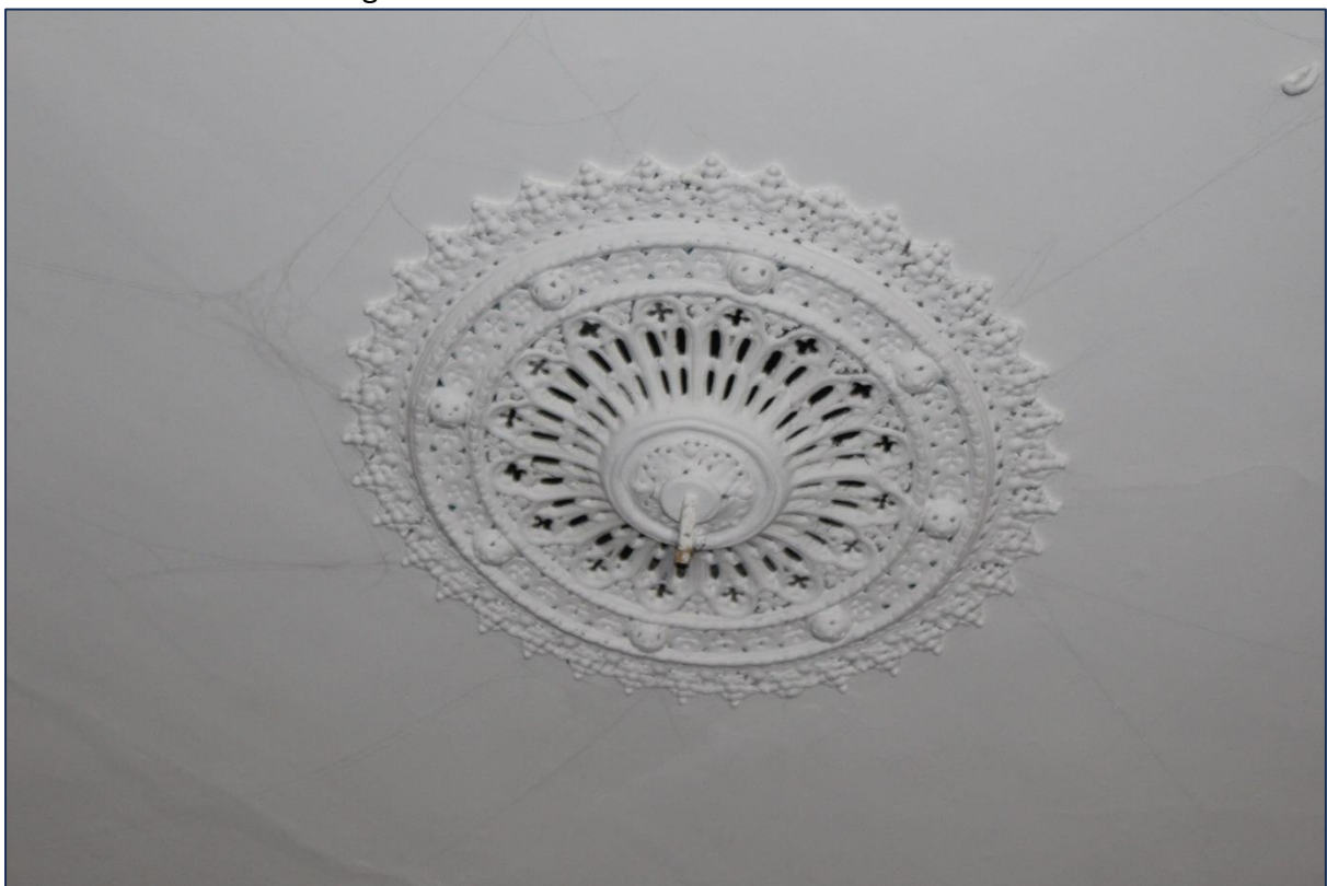
Plate 29: Decorative ceiling rose in exercise hall.
