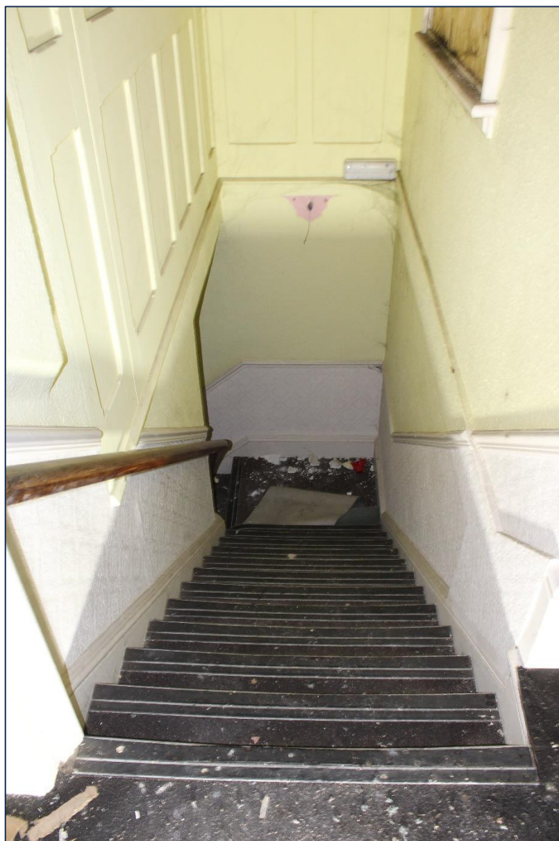
Plate 32: Stairwell to entrance hall looking northeast.
