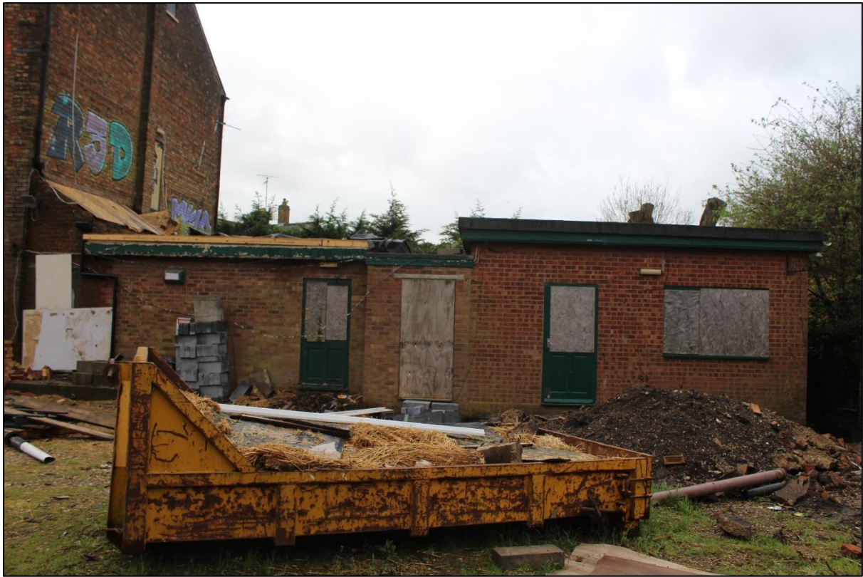
Plate 6: northeast elevation showing postwar extension to building.
