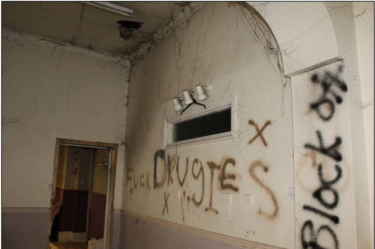
Plate 8: Exercise room looking south.
