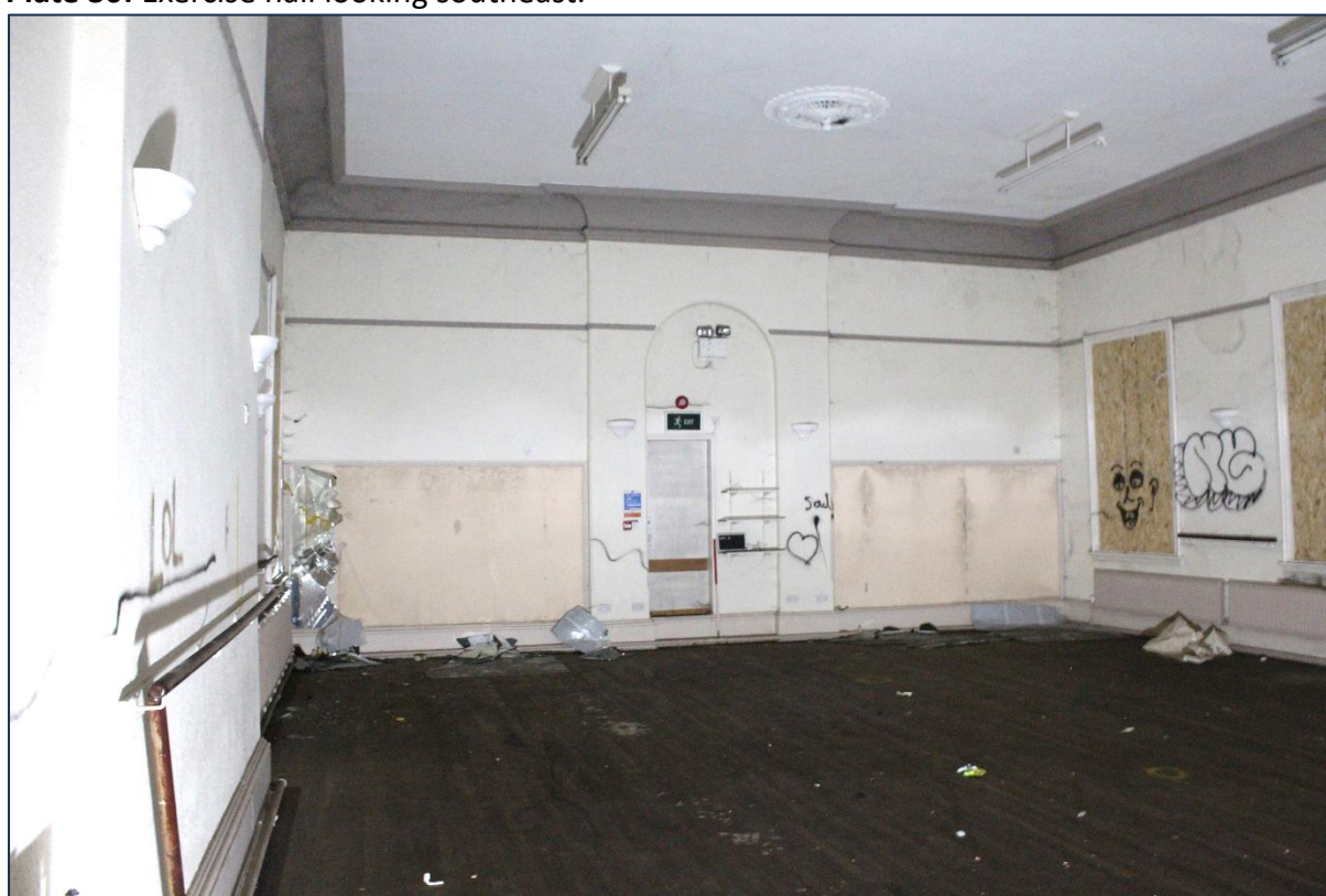
Plate 31: Exercise hall looking north.
