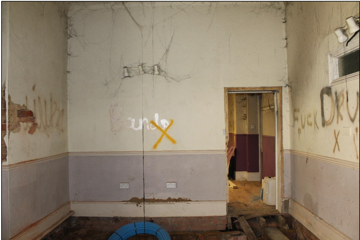
Plate 10: Exercise room looking south.
