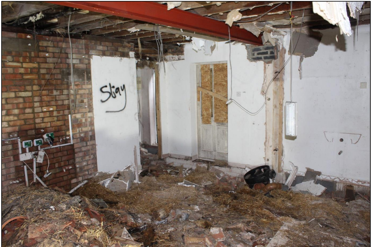
Plate 26: Store B, store C and boiler room looking north.
