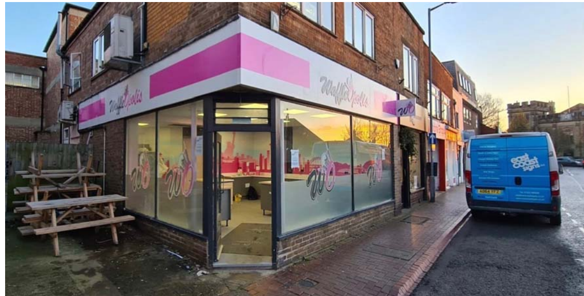
Photograph of North-West Elevation
