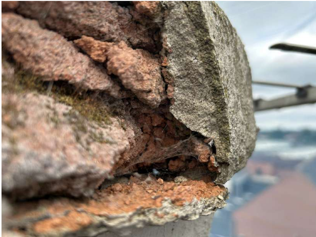
Photo 03 - Existing Chimney close detail
