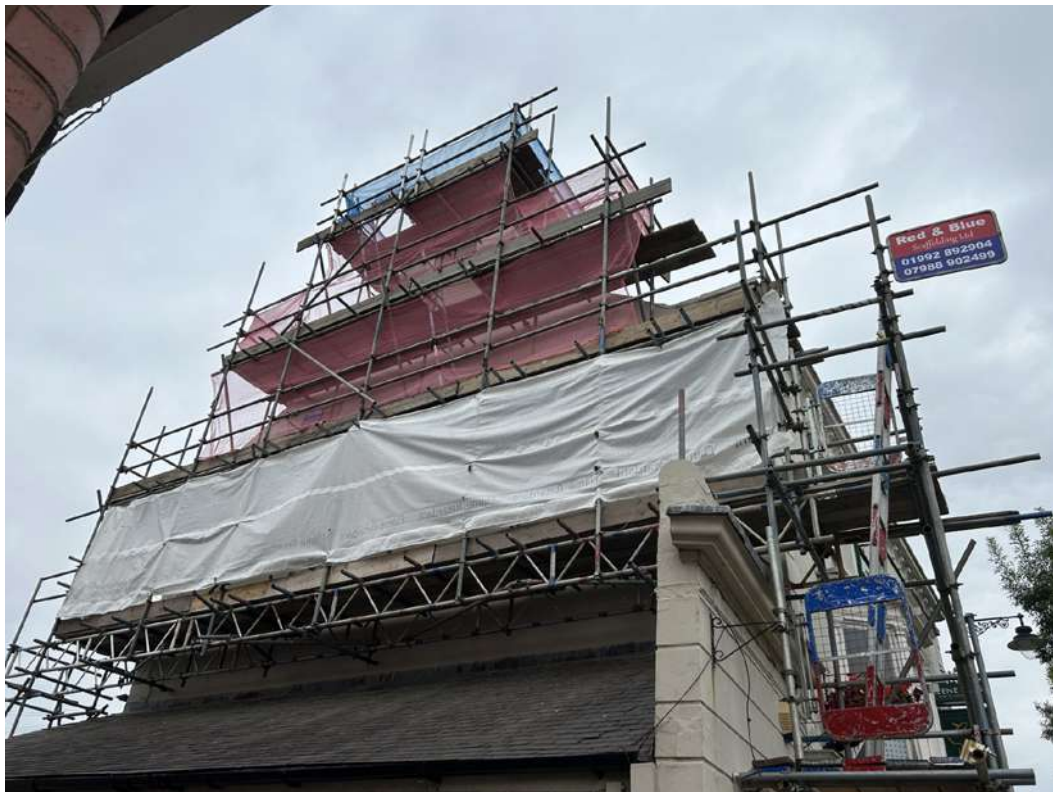
Photo 01 - Existing Side view
