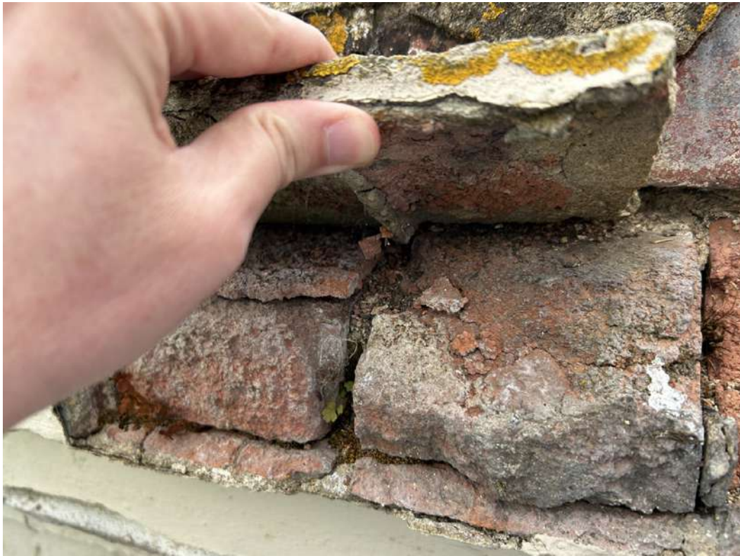
Photo 04 - Existing Chimney close detail
