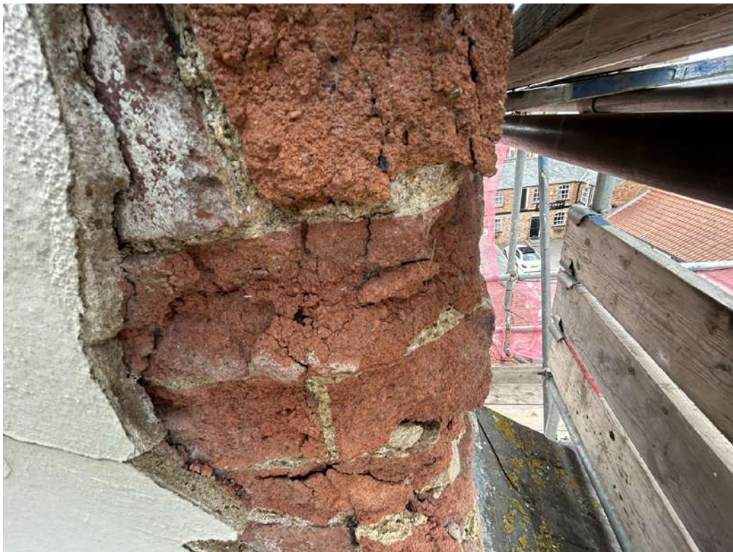
Photo 02 - Existing Chimney close detail
