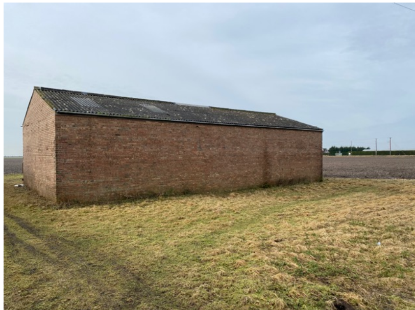
View from the road, looking north-west
