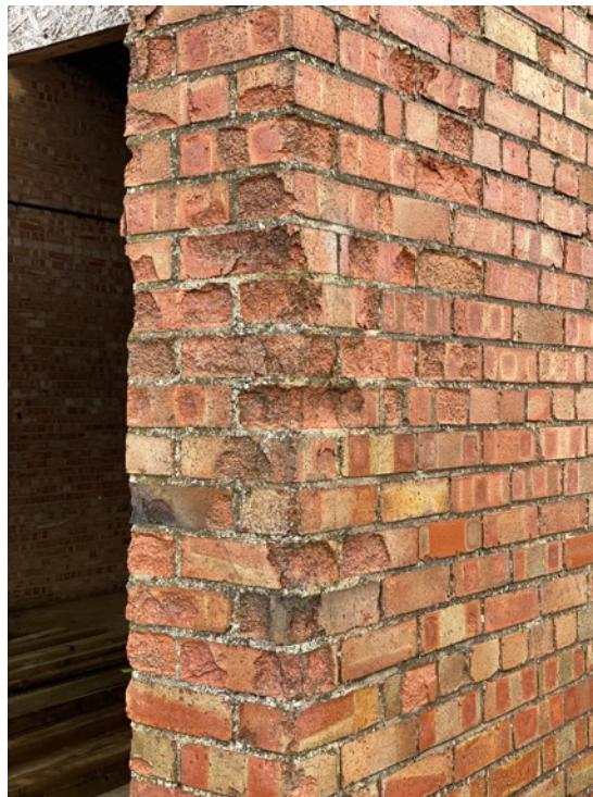
The south west corner
