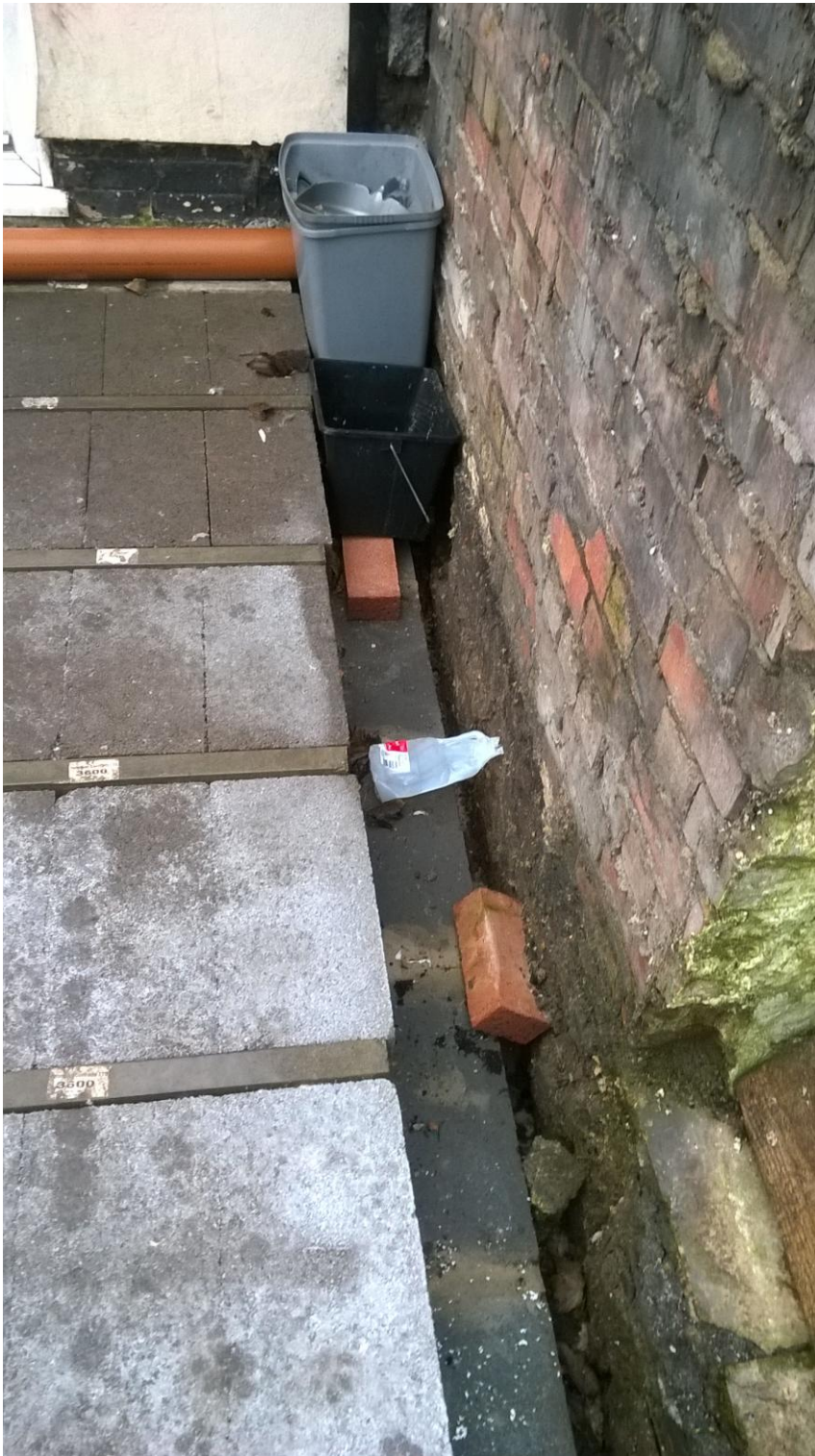
Beam and block floor at boundary wall location
