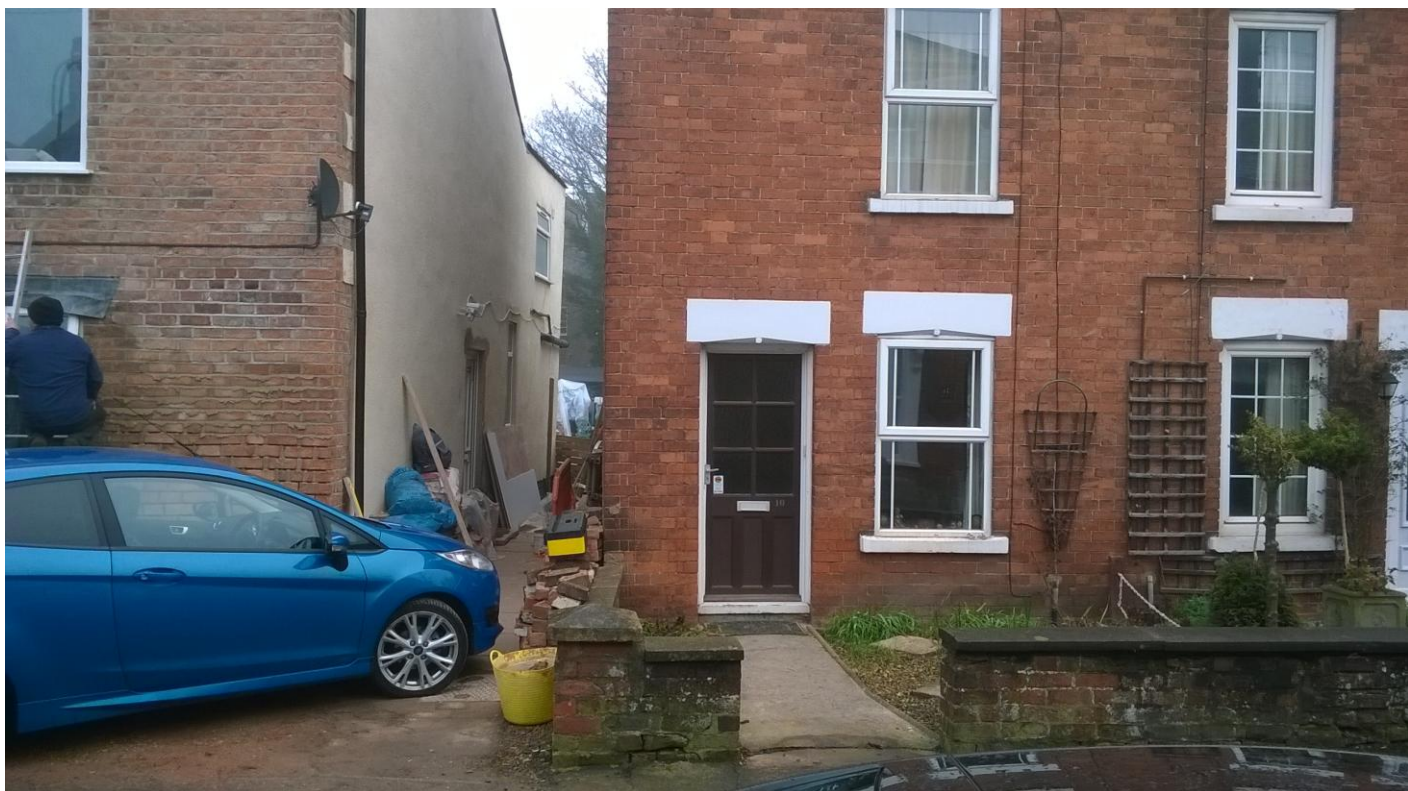
View from front showing access to side of property
