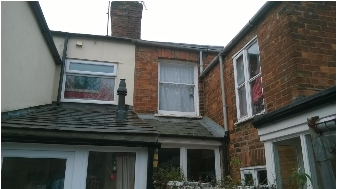
Rear elevation of numbers 8 and 9 at boundary wall position
