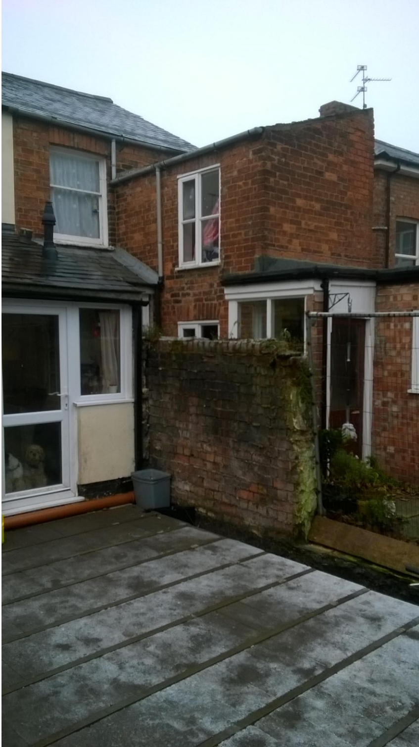
View of beam and block suspended ground floor construction of the proposed Extension and across the boundary wall to number 8
