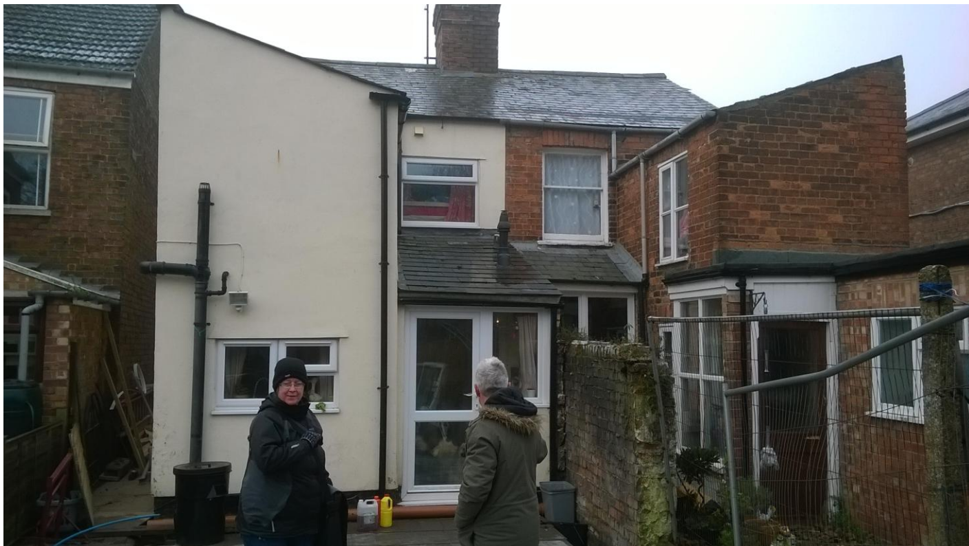
Wider shot of rear elevation
