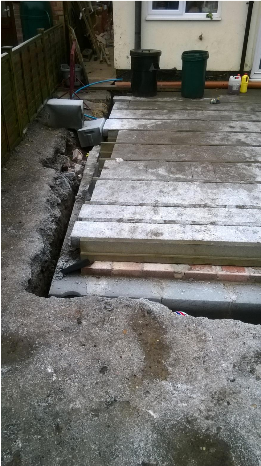
Beam and block suspended ground floor construction
