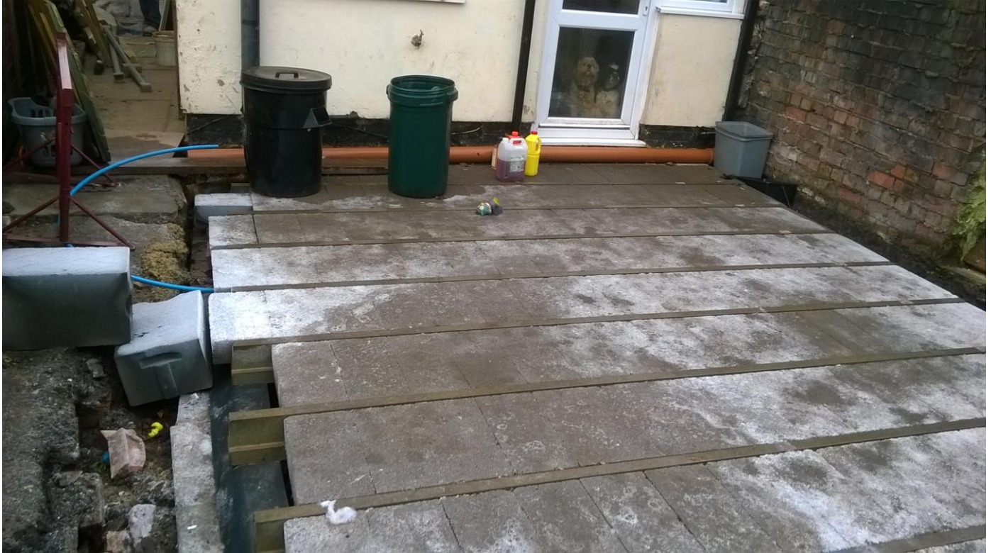
Beam and block suspended ground floor construction in progress
