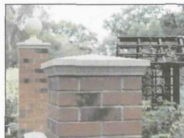
SCA28 pier cap
