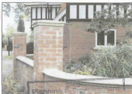
Special radius coping & SCA28 Pier caps
