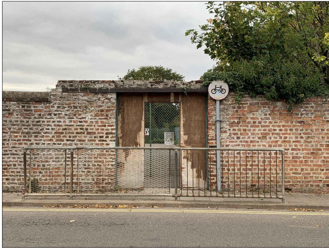
View of gate from east (Love Lane)
