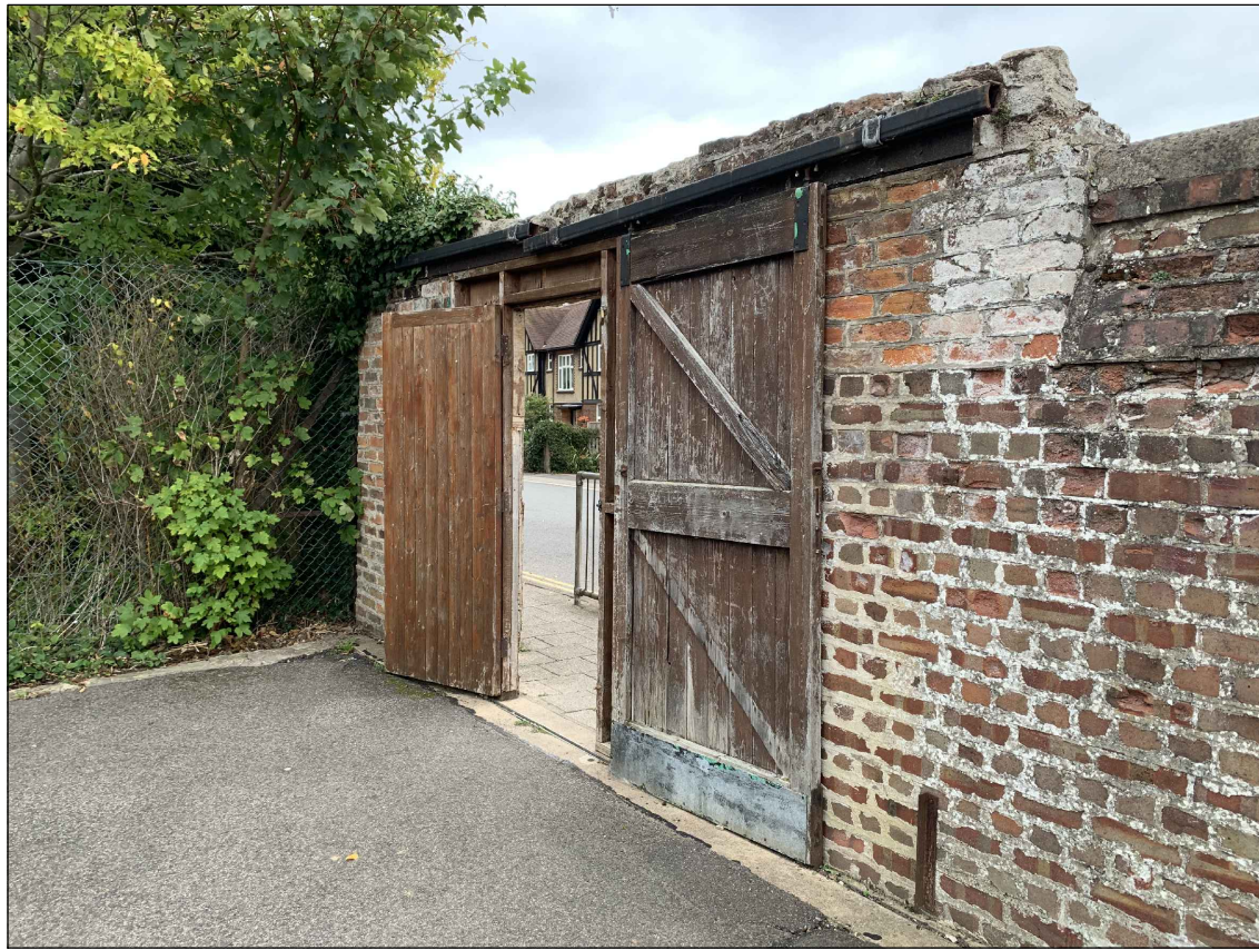
View of gate from west (Ayscoughfee Hall Gardens)
