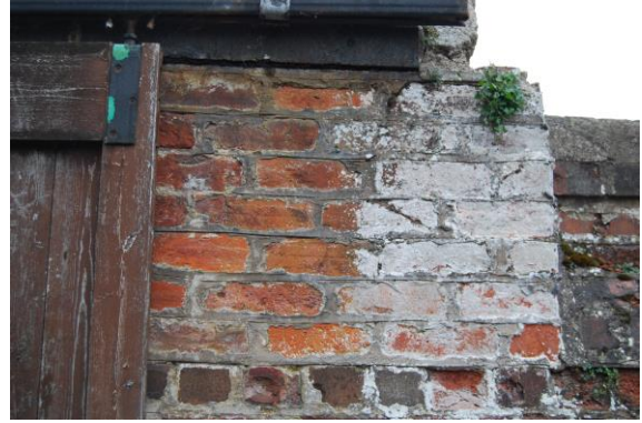
Fig 11. Photographs to either side of the opening showing where original brickwork has been replaced
