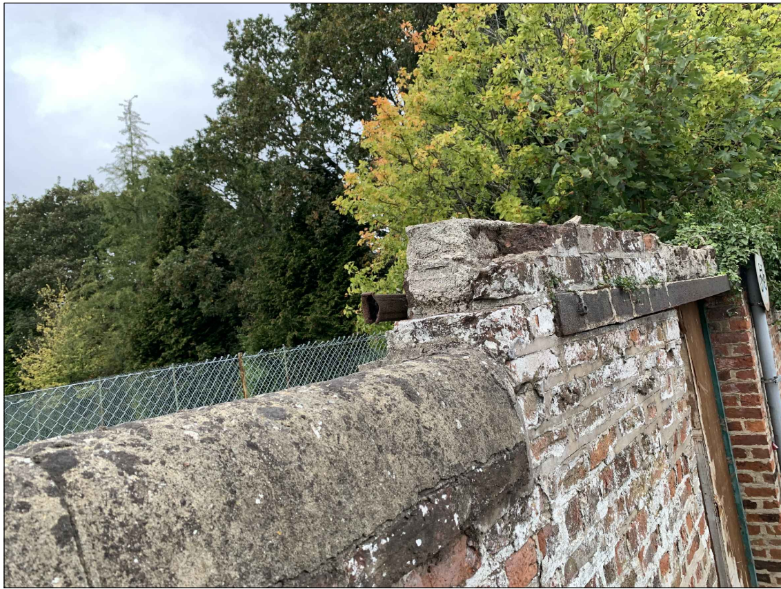
Rendered half round capping detail
