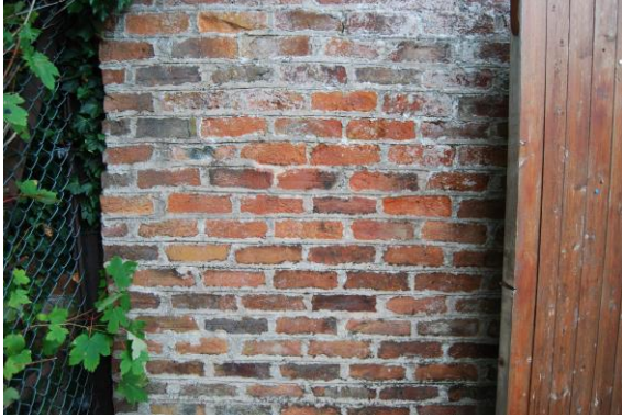
Fig 11. Photographs to either side of the opening showing where original brickwork has been replaced
