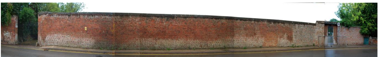
Fig.2 Panoramic view of the boundary wall and gates in Love Lane
