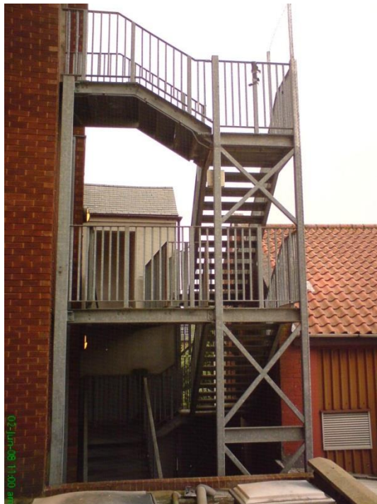
South Holland Centre fire escape stair from flat roof to rear of 24, Market place
