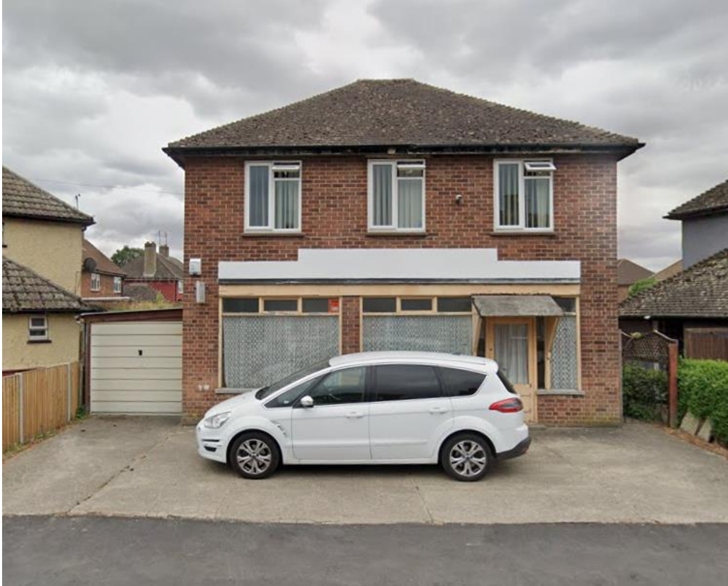
View from east side of site
