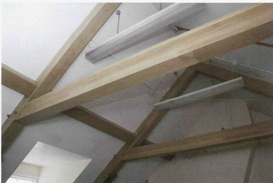
Plate 6: Holland House – modern replacement laminated truss roof structure
