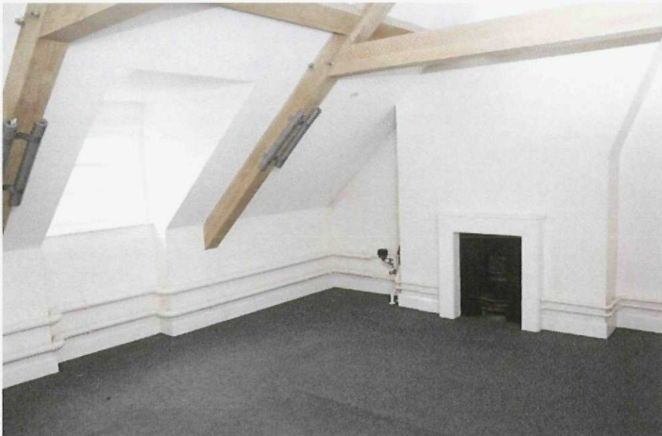
Plate 4: Holland House – front second floor room on the north-eastern side of the building
