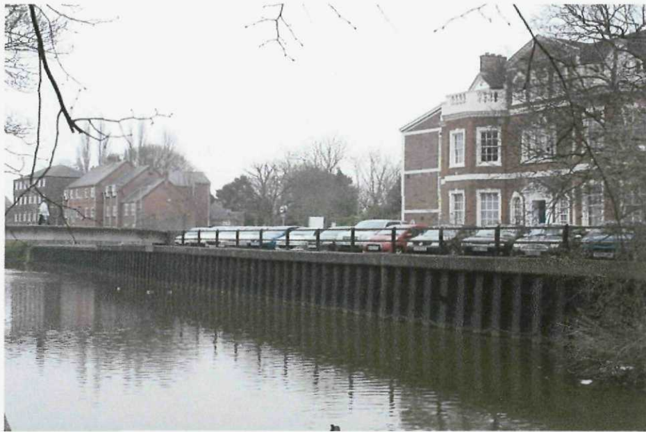
Plate 6: The break in the enclosure of High Street to the north-east of Holland House and the group of riverside buildings beyond, including the grade II listed Star Relay Warehouse
