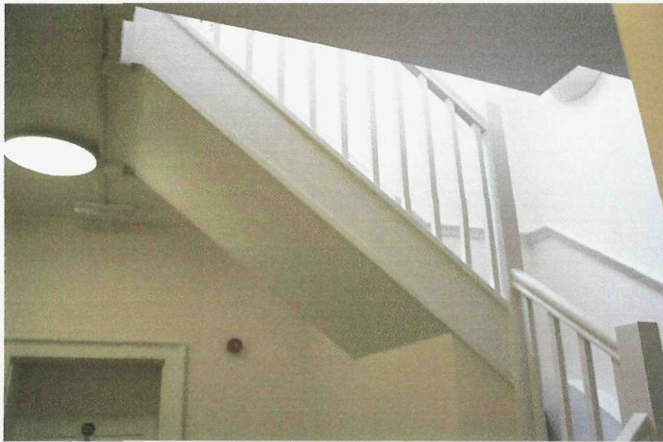
Plate 26: New secondary staircase from first to second floor
