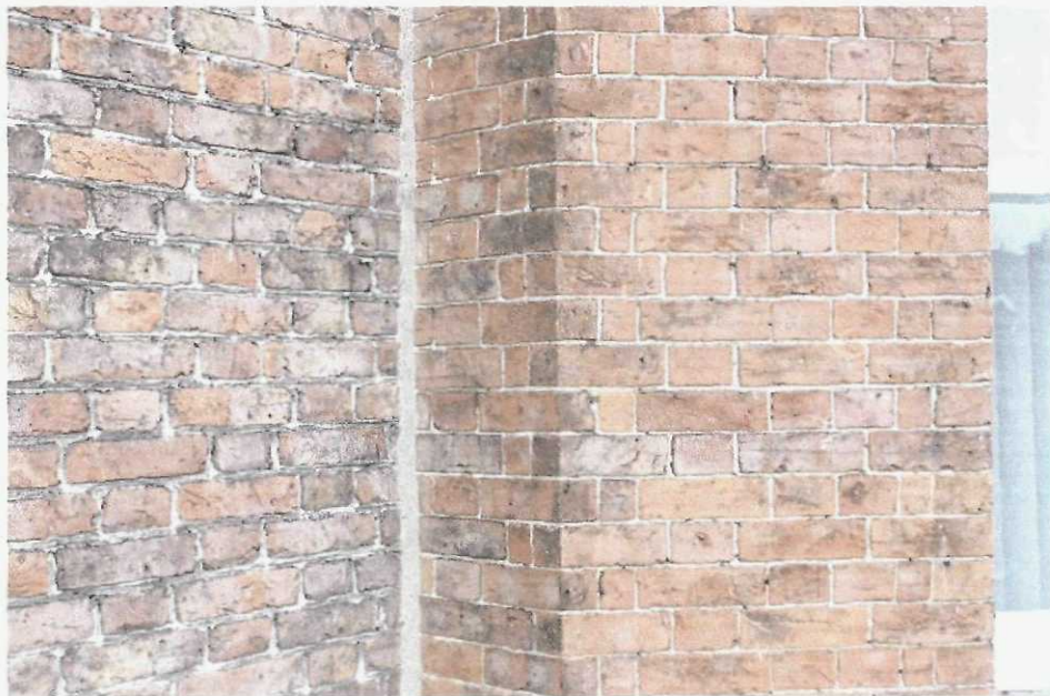
Plate 12: Original 1760s brickwork to the left and later Georgian/early Victorian brickwork of the rear facade canted bay to the right
