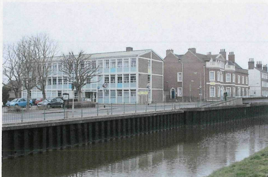
Plate 5: The Government Offices building built in 1960 and the car park to its north-east
