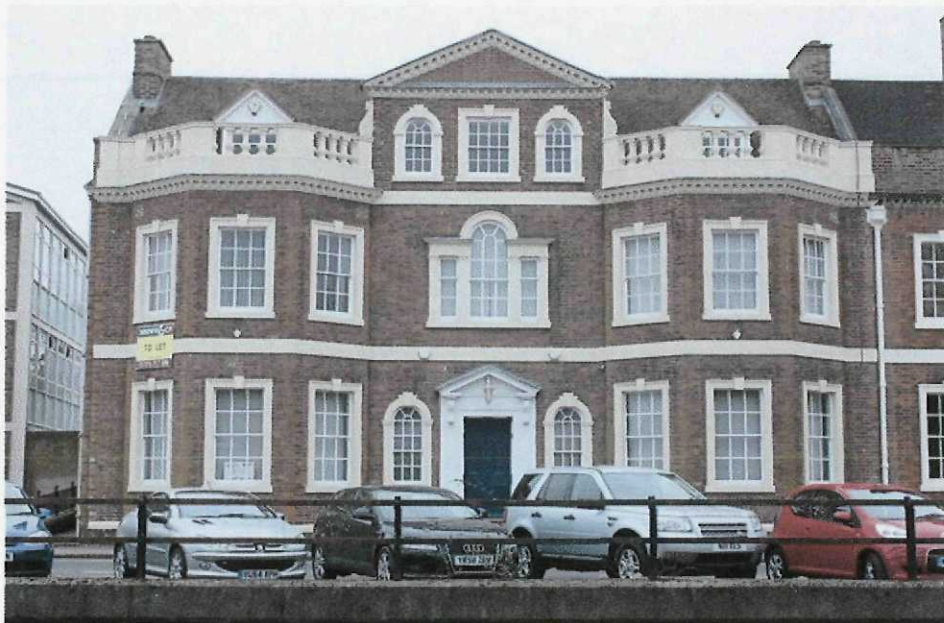
Plate 8: Holland House – the principal north-west-facing High Street facade
