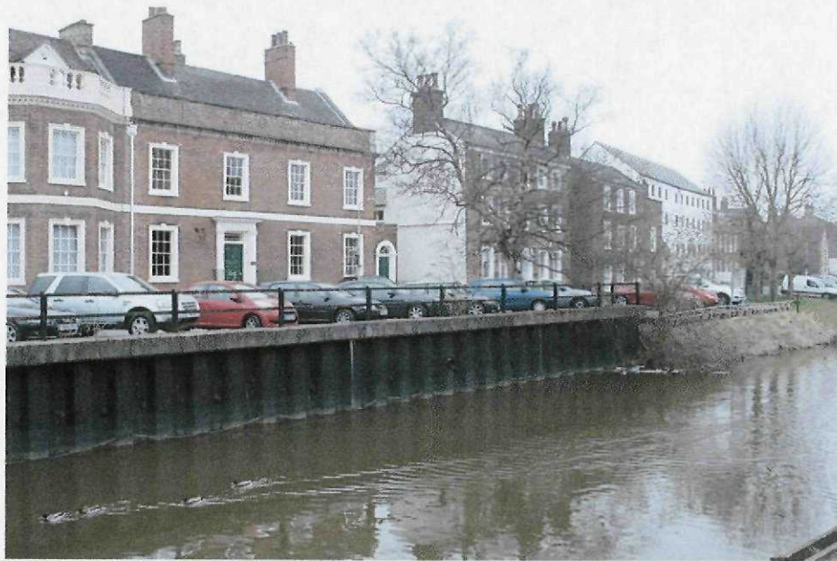
Plate 4: No.16 High Street and a group of former merchant's houses and warehouses beyond
