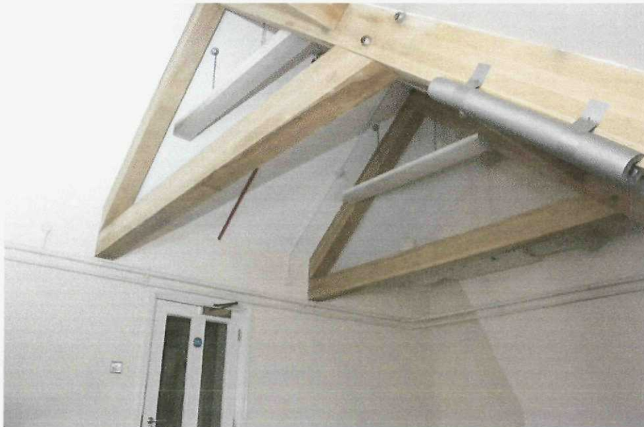
Plate 30: modern replacement laminated truss roof structure
