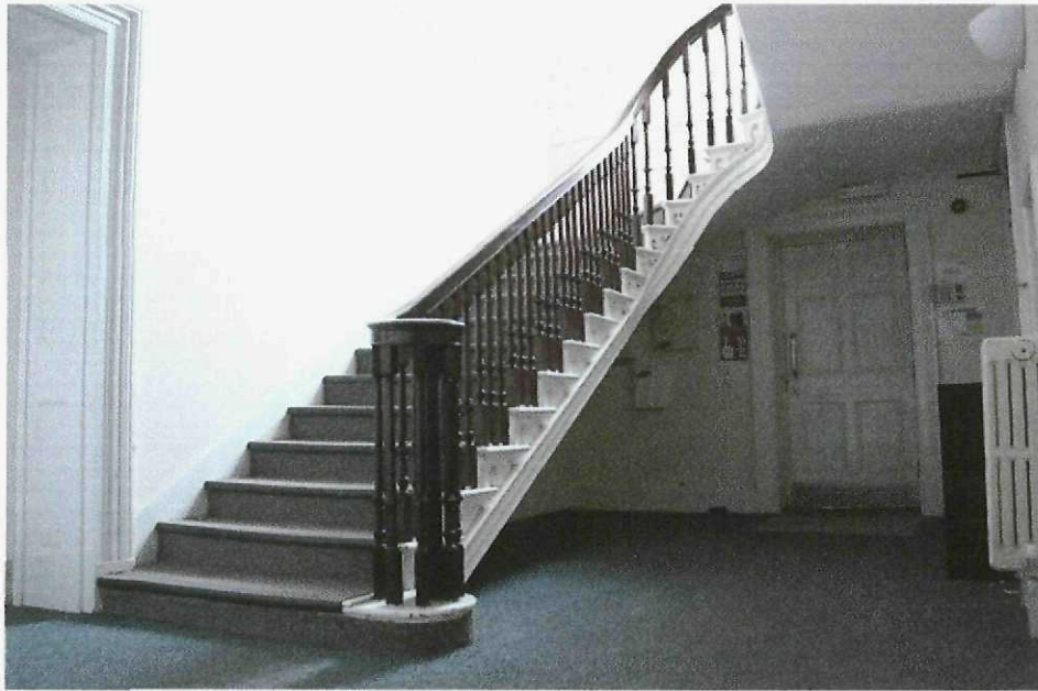
Plate 16: The restored cantilevered cut-string timber staircase
