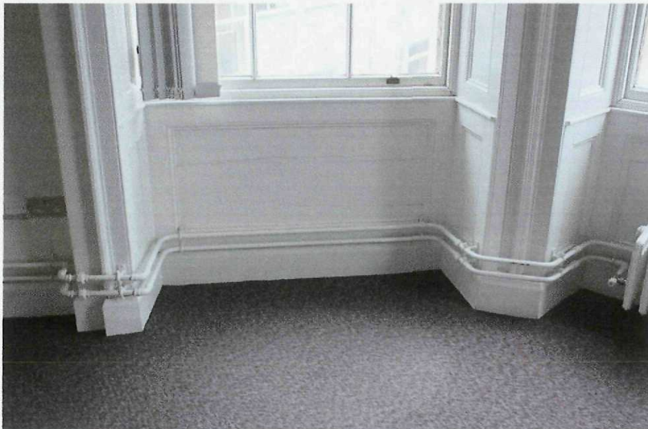
Plate 29: Original panelling to rear first floor canted bay
