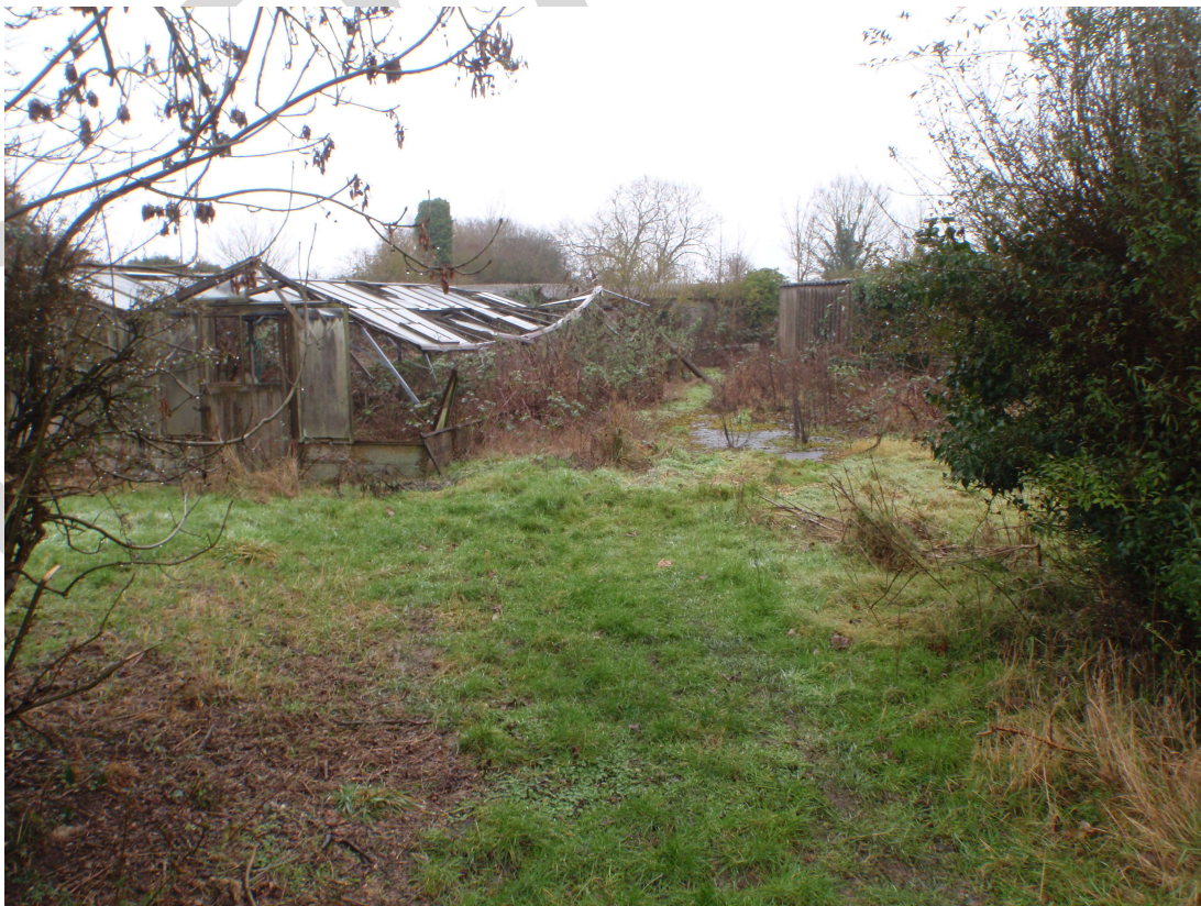
Plate 2: View of structure in the northern part of the site (obstructing the proposed location of Trench 4), looking south.
