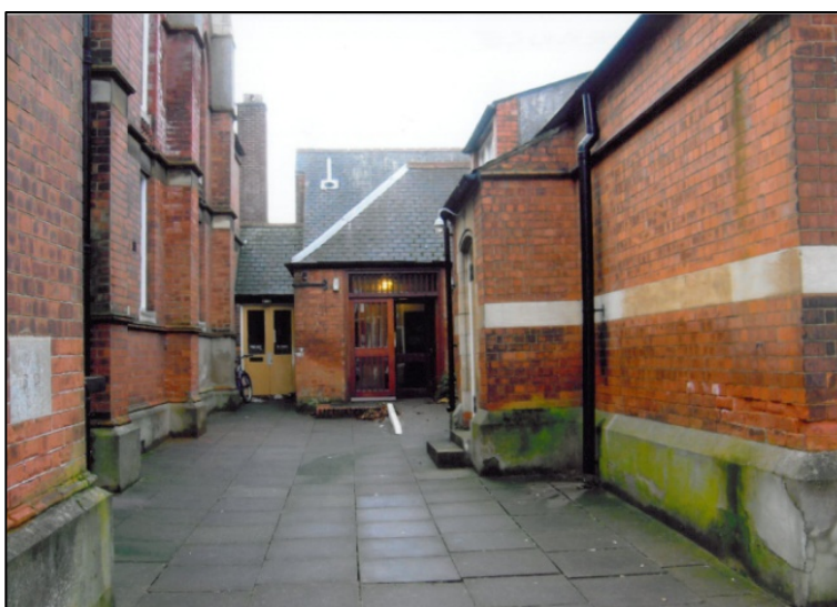
External space between church and hall
