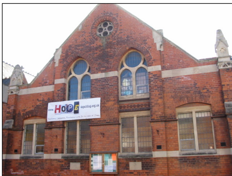
Front façade of hall (Sunday School)
