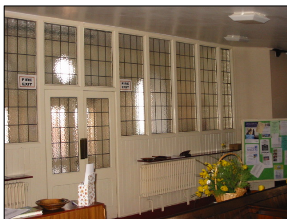
Glazed screen to vestibule
