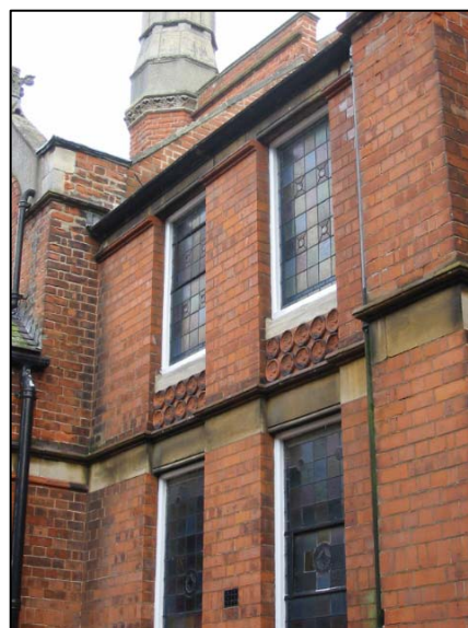
View of side façade (North West)
