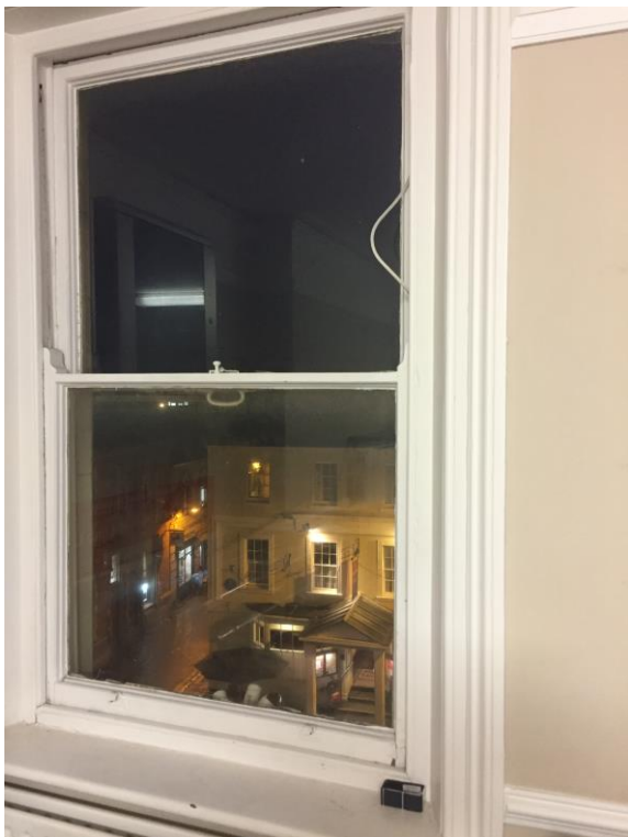
Fig. 32 North window with horns visible
