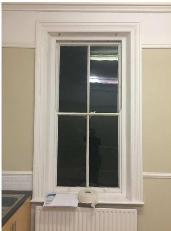
Fig. 33 South window with lamb's tongue glazing bars
