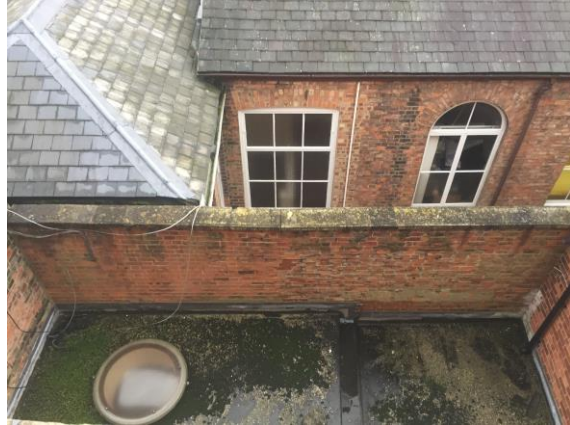
Fig. 05 Abutting building to rear (south-west).
