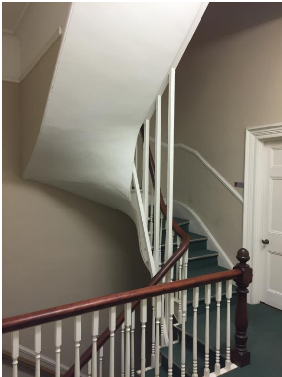
Fig. 18 Stair from first to second floor level
