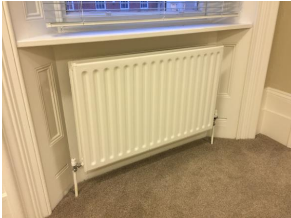
Fig. 26 Window recess in Room F1.
