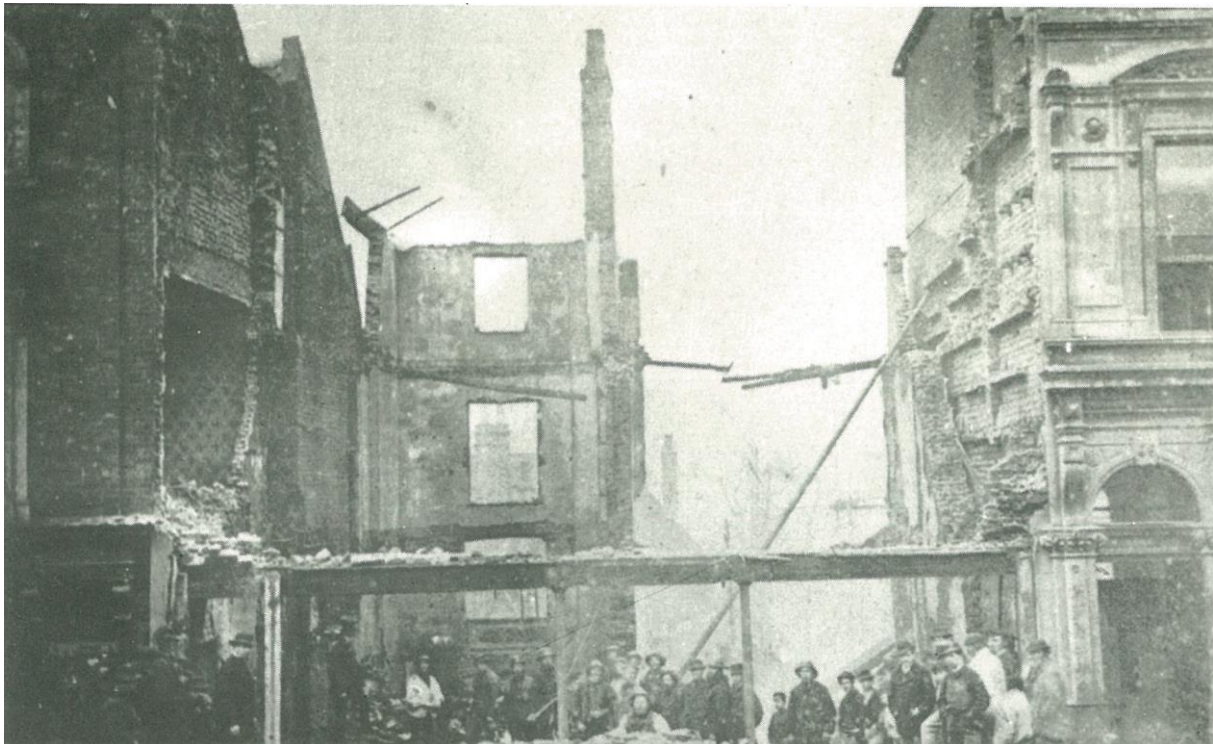
Fig. 15 Photograph taken after 27 th March 1870 following the fire at Hobsons – site on extreme right.
