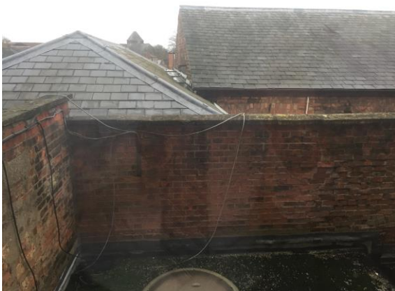
Fig. 06 View at FFL to south-west into enclosed lightwell.
