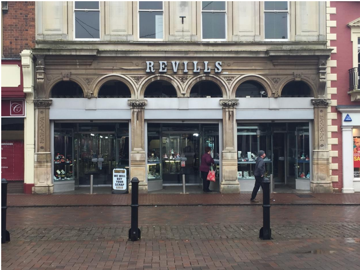
Fig. 17 The north-east elevation at ground floor level as it exists in 2017.
