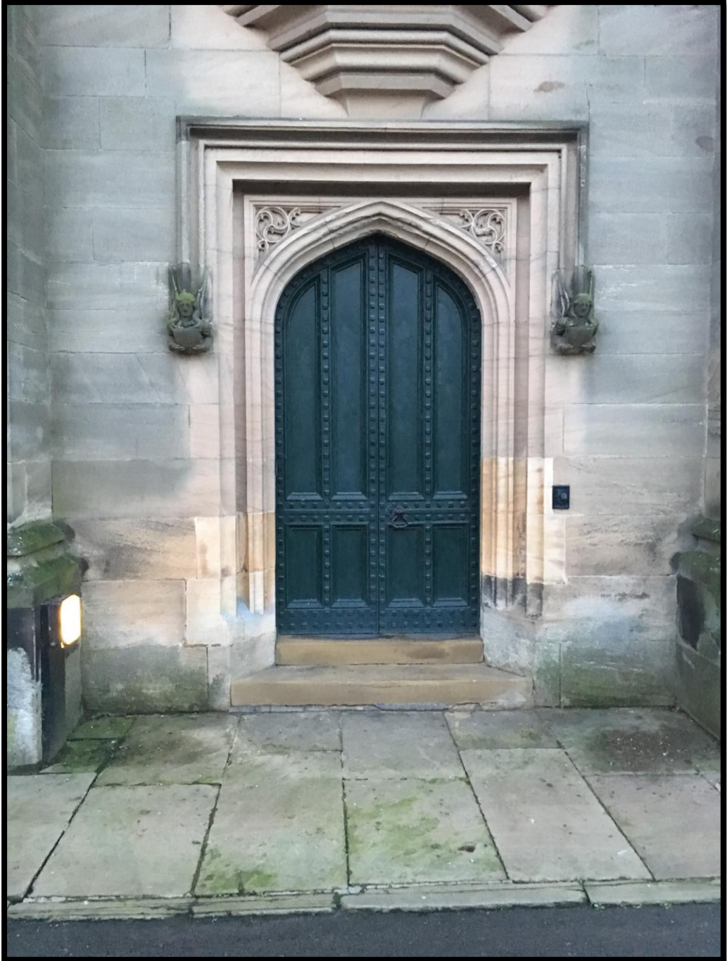
Example of existing doorway with external light
