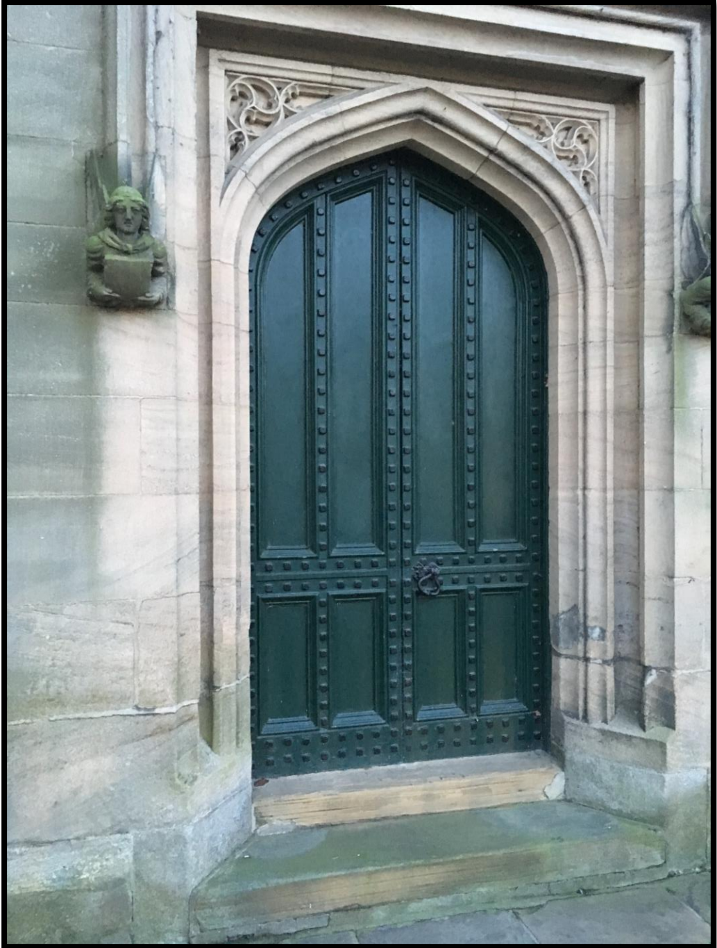
Position of new doorbell
