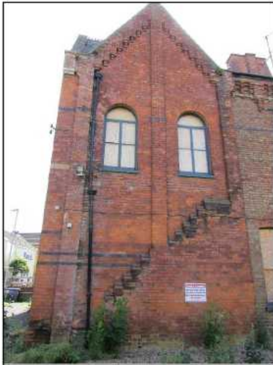
Figure 5 - Close-up detail of North elevation.
