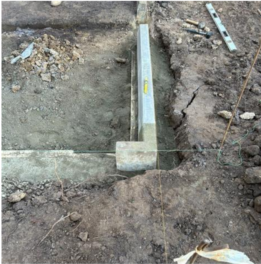
Kerb corner and setting out
