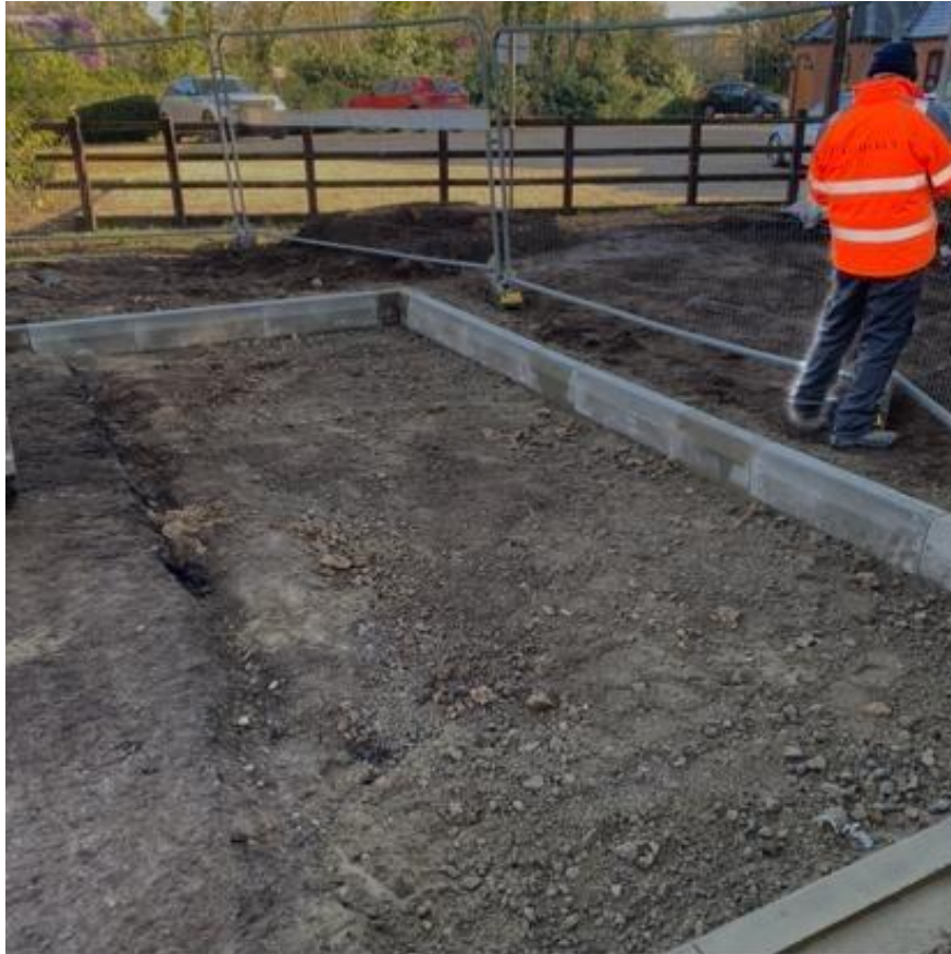
Kerbs complete ready for final prep for tarmac on Monday
