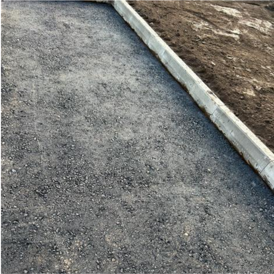
Base tarmac laid
