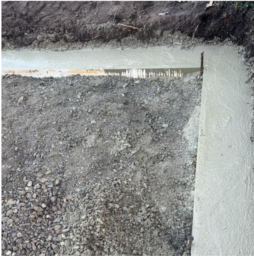
Kerb race laid
