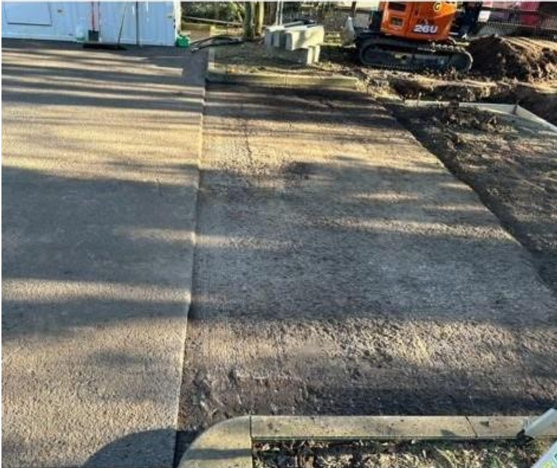
Planed edge tidied up ready for tarmac
