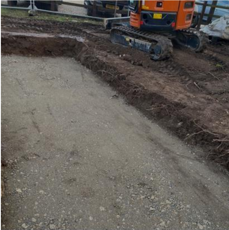
MOT Type 1 sub-base laid and compacted
