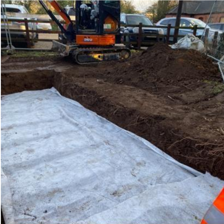
Geotextile membrane laid prior to MOT Type 1
