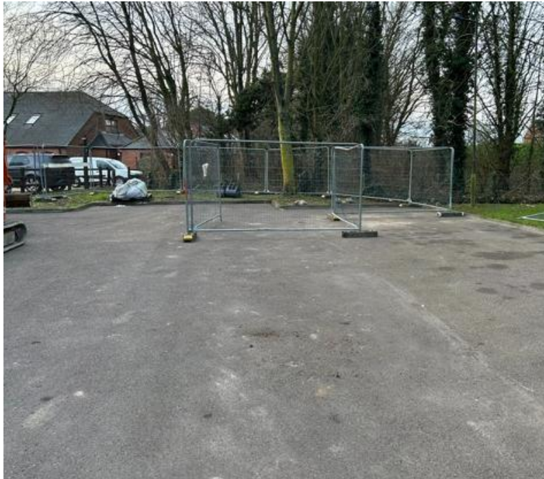
Site Set Up
