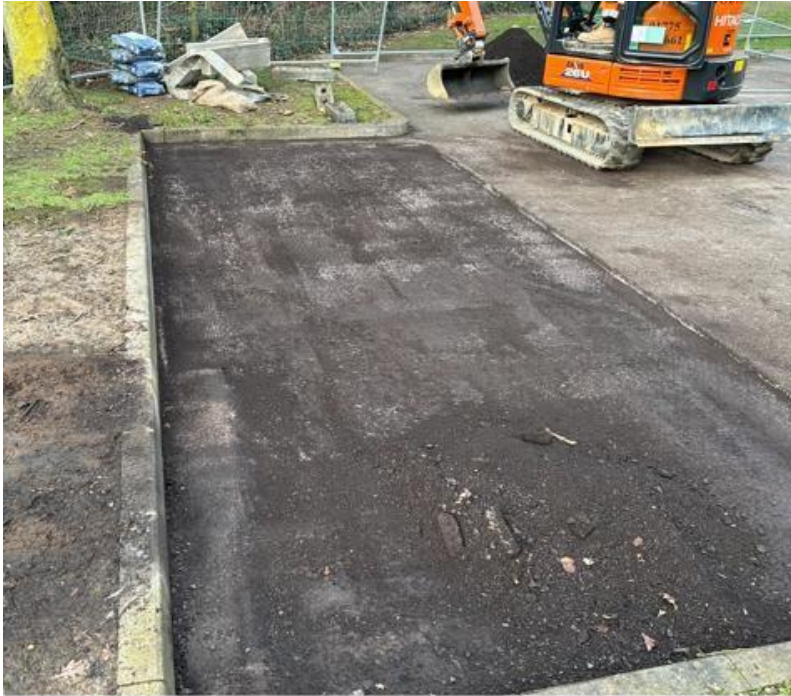
Planing works completed
