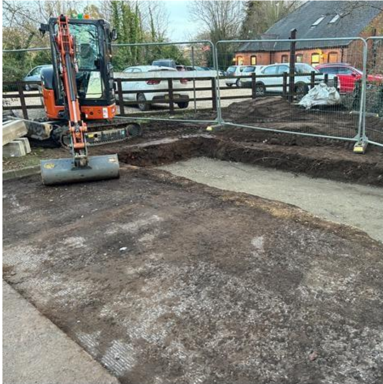
End of day, ready for kerbing works
