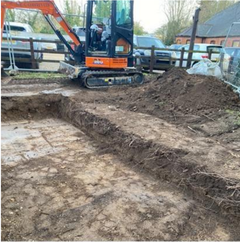
Excavated to reduced levels
