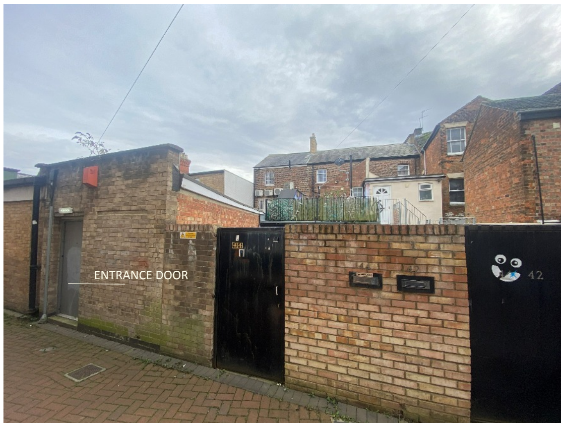
VIEW FROM CHAPEL LANE TO THE REAR ENTRANCE / EXIT
