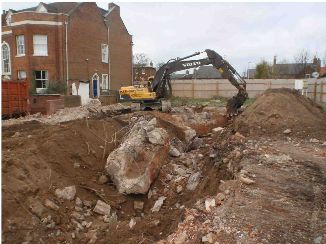
Plate 4. Removing concrete foundations looking northwest
