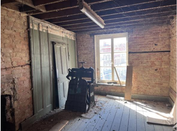
Fig 04. Disused room at upper level.
