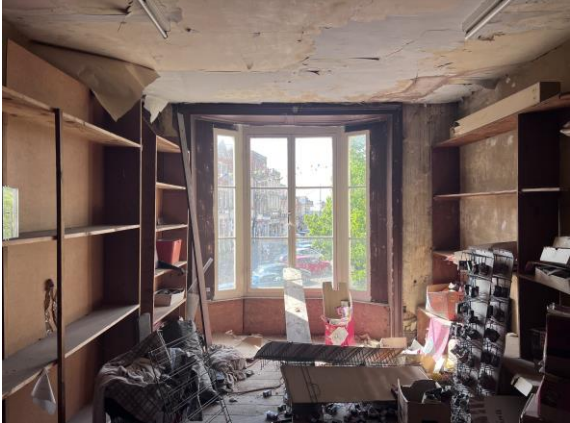
Fig 05. Disused room at upper level.
