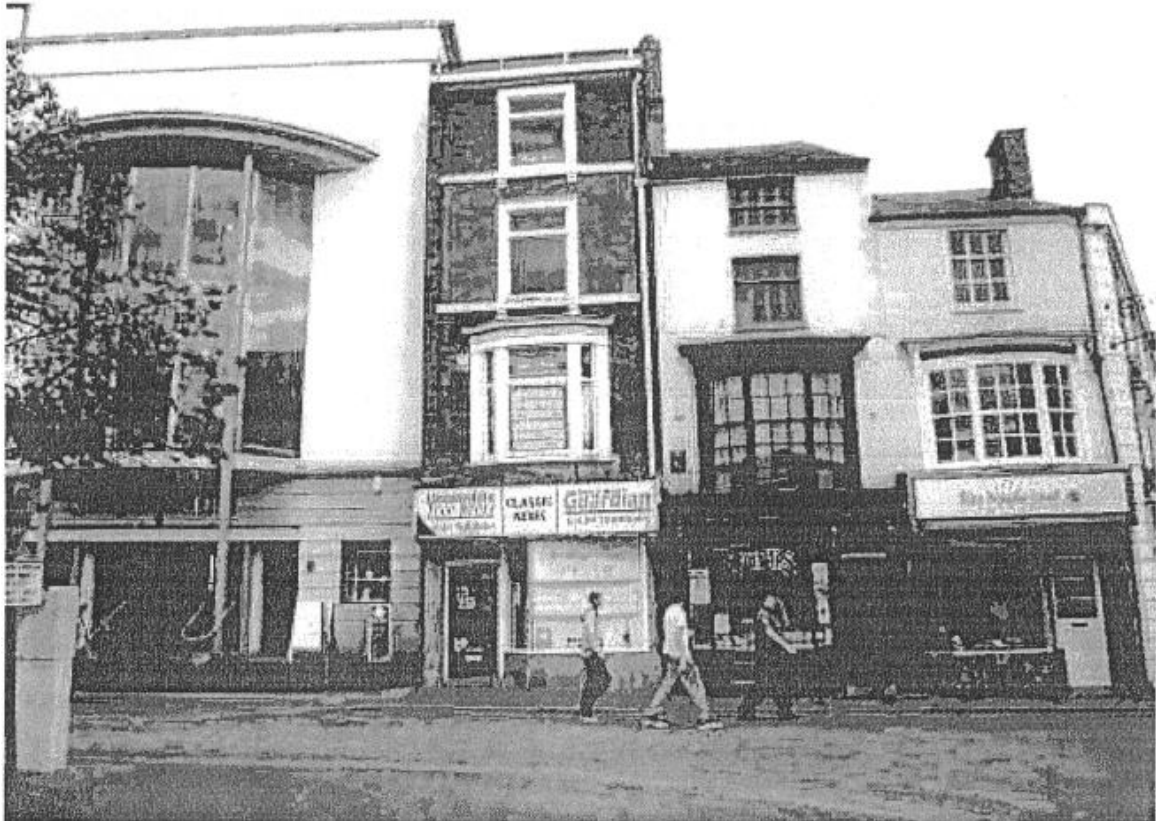
Fig 18. Image from 2011 prior to the most recent remodelling.
