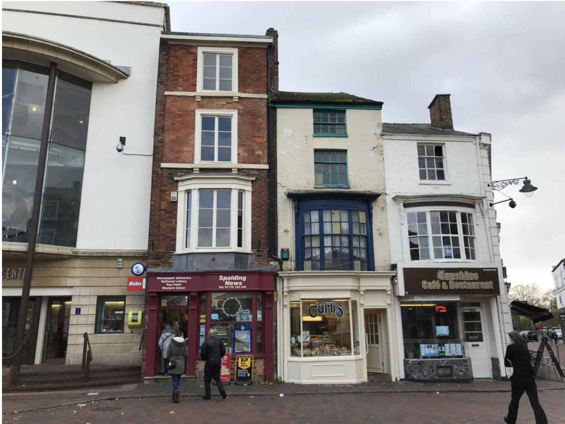
Fig 19. Image as the building exists in 2025.
