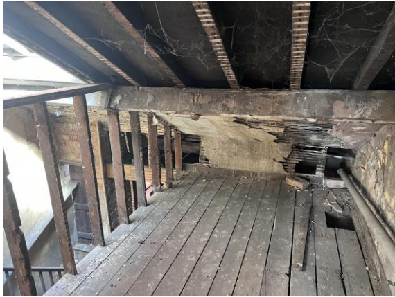
Fig 06. Disused area at upper level.
