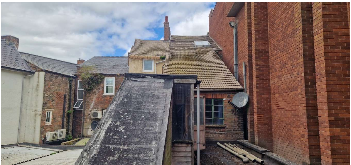
Rear elevation from flat roof
