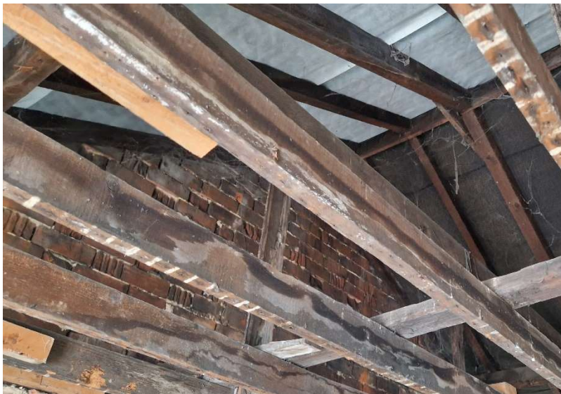
General internal views of roof
