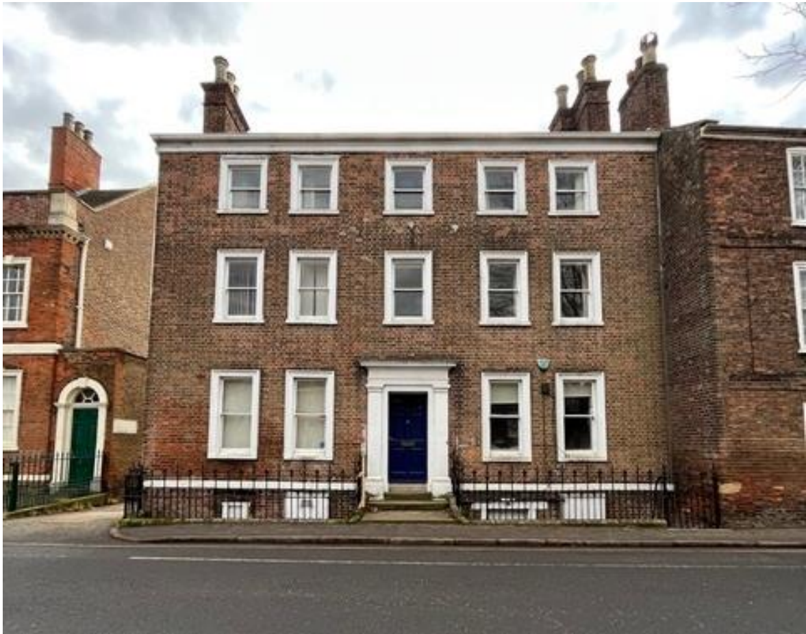
View of existing building
