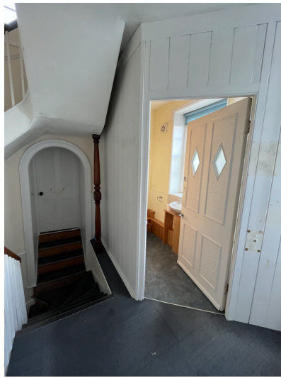
p5. partition wall to be removed
