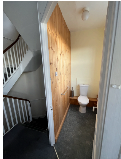
p6. partition wall to be removed
