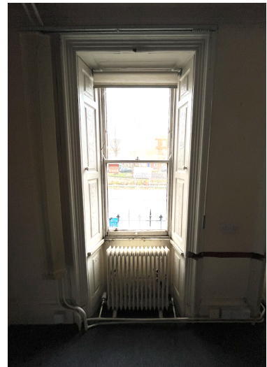
p3. Window frames to remain
