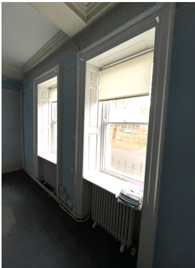
p1. Window frames to remain
