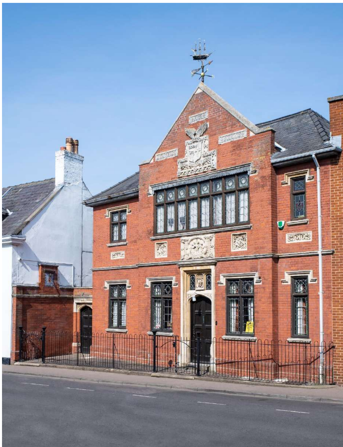
A PHOTOGRAPHIC BUILDING RECORD OF THE MUSEUM OF THE SPALDING GENTLEMEN'S SOCIETY IN RELATION TO DEMOLITION WORK APPROVED BY SOUTH HOLLAND DISTRICT PLANNING REFERENCE: H16-0932-22
