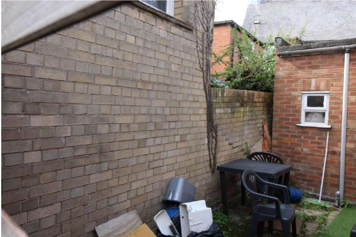
Rear of barber's shop showing exterior of Maples Room and the wall between numbers 8 & 9
