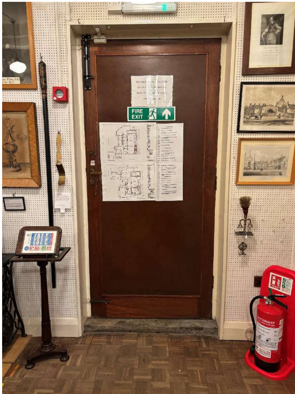
External door/fire exit
