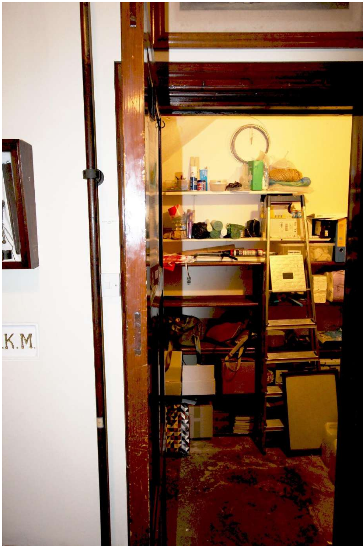
Outward-opening door and interior of store cupboard
