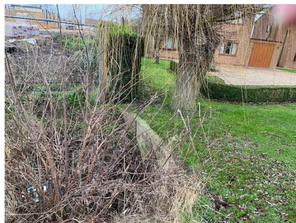
Frontage Ditch / Headwall at northern boundary
