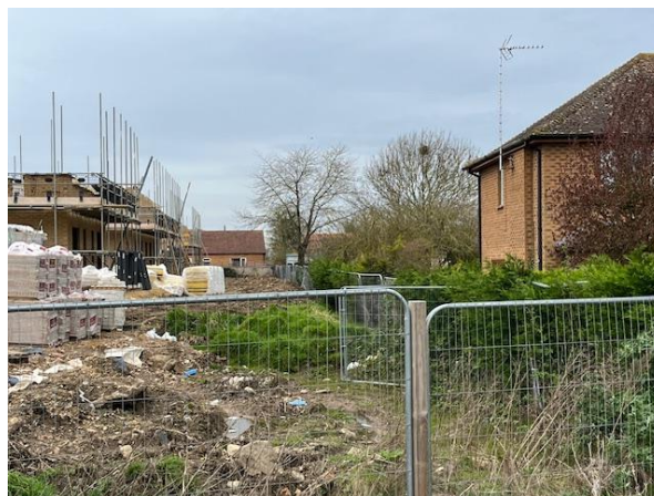
New Development under construction behind application site
