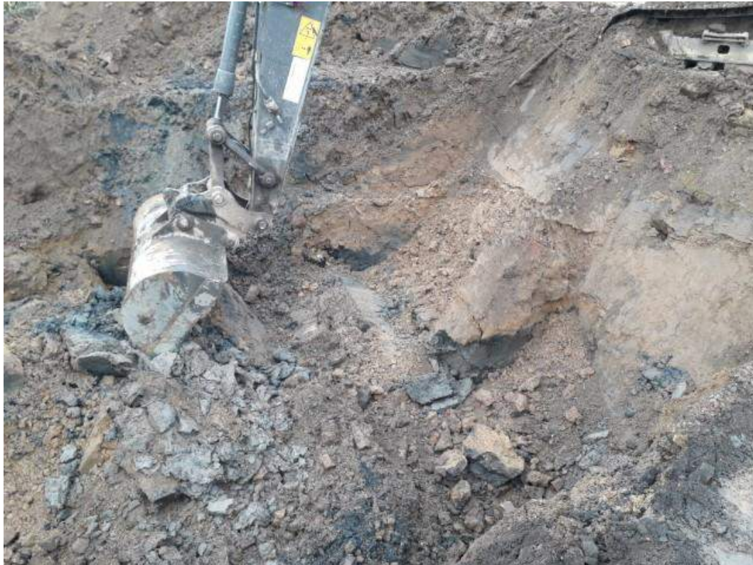
Extension of excavation east to locate cradle wall on the eastern side of the tanks. It was concluded that there were only three sides remaining to the cradle. The wall along the eastern side was not proven.
