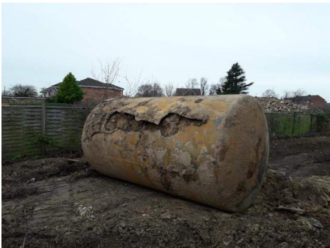
As above. Sand/cement slurry fill can be seen inside the tank.
