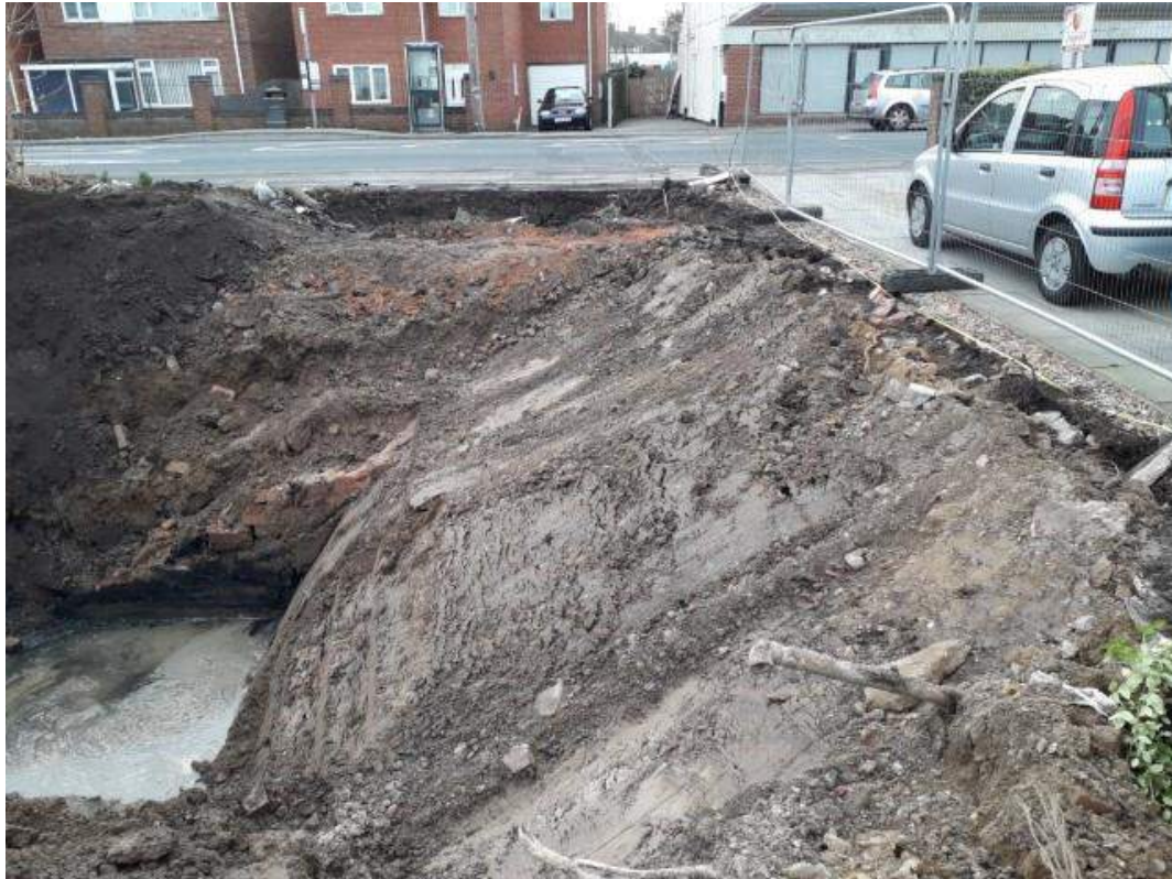
Western face of excavation. Note batter for stability to ensure driveway was supported.
