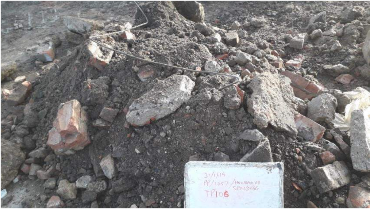
TP106, made ground spoil (former floor slab/foundations).
