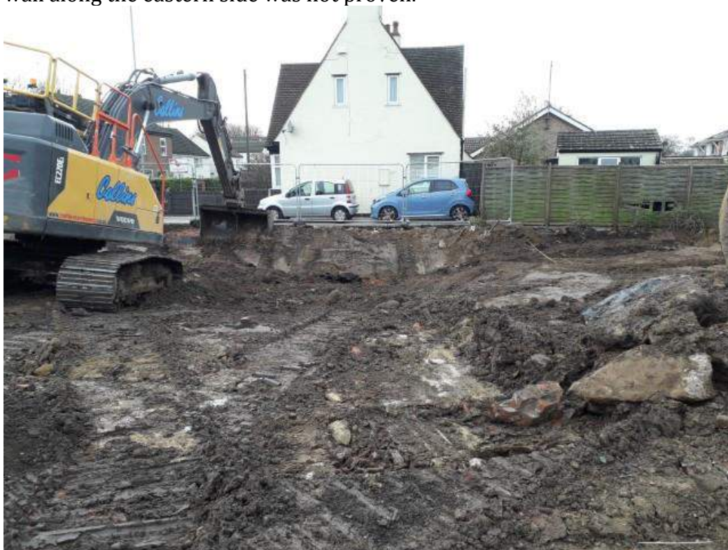
Backfilling cradle for safety reasons. View west towards adjacent dwelling.
