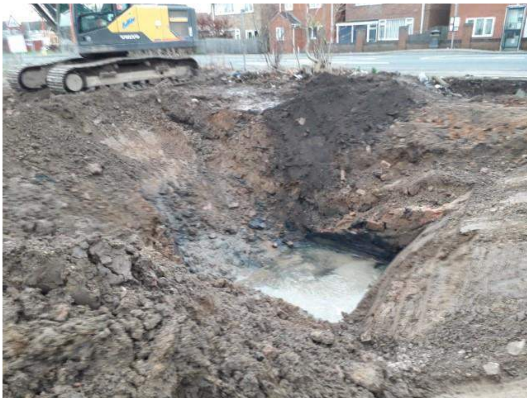
Looking south-east from north-west corner. Note water trapped/ponded on the concrete at the base of the excavation. The water was around 100mm deep in places.
