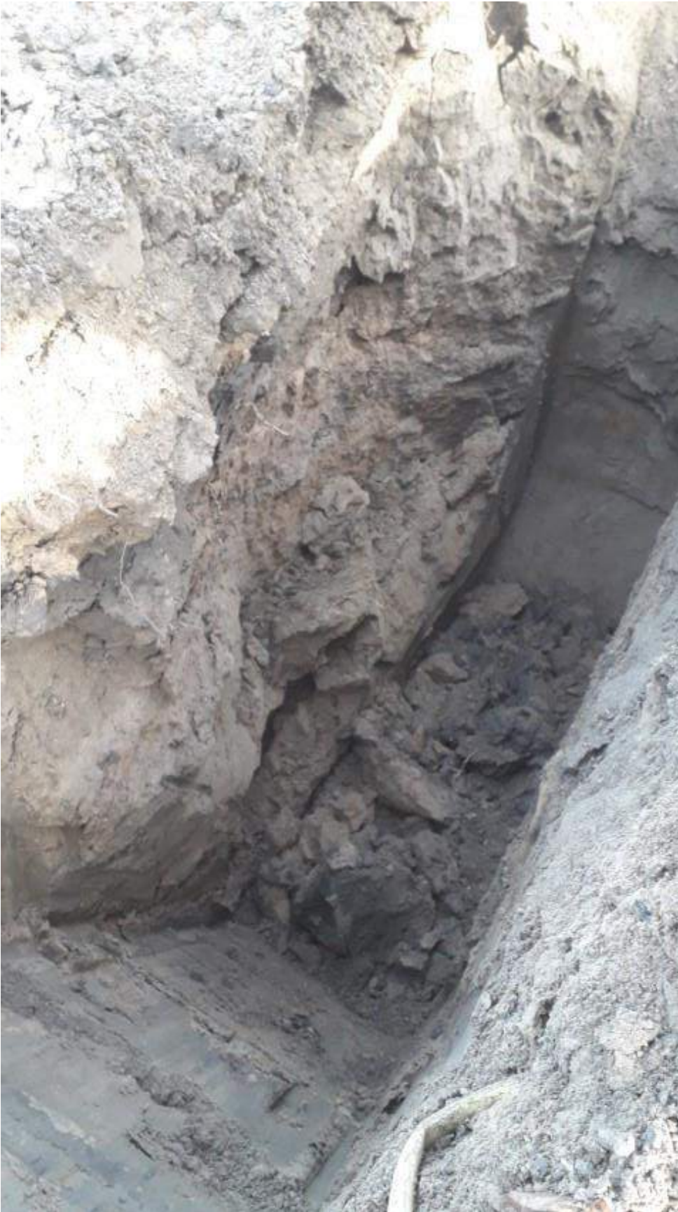
TP107, showing some spalling of sides.
