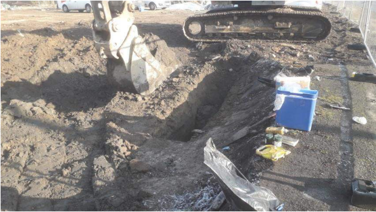
General view east showing TP103 excavation.
