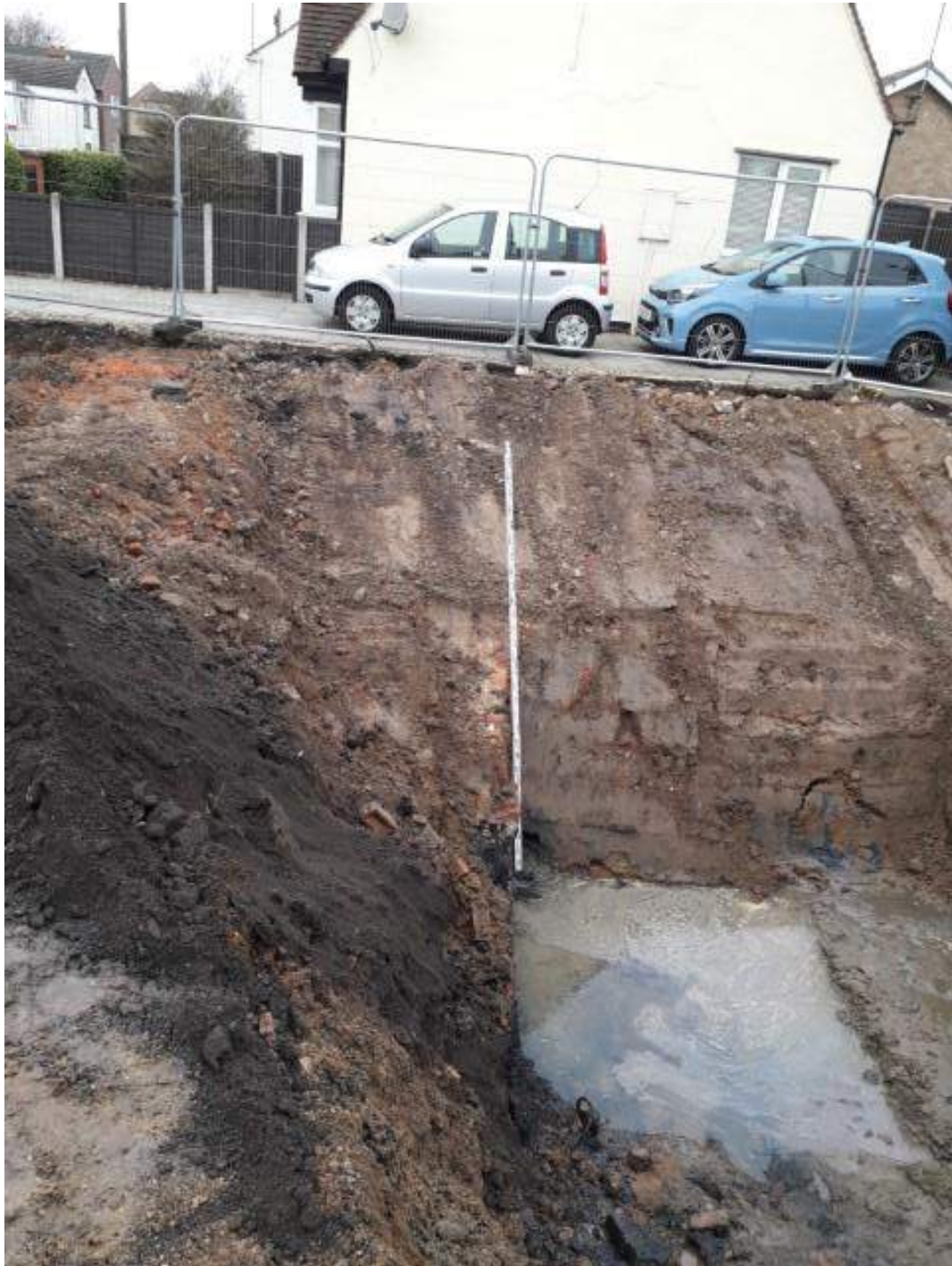
Survey staff lowered into the excavation to measure depth of excavation. Looking west across excavation. The concrete base is approximately 2.40m below original ground level.
