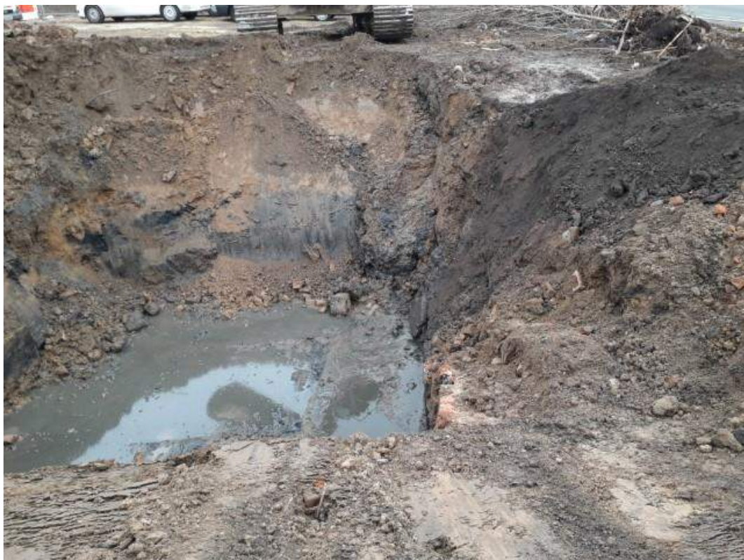
View looking west across cradle excavation.
