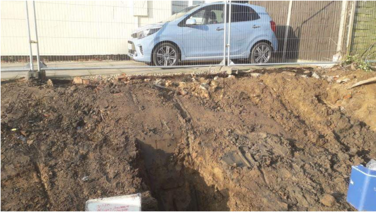
TP101, within batter adjacent to driveway of residential property to the west.
