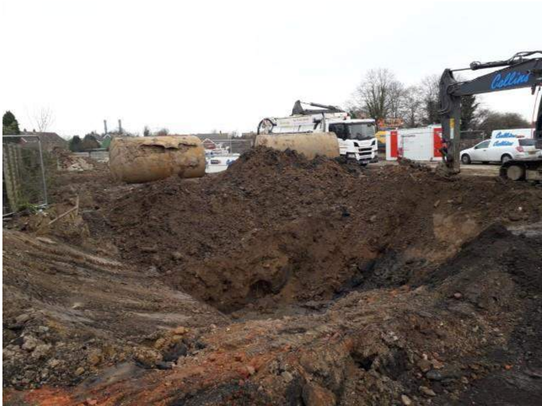
Soil with no visual or olfactory evidence of impact from upper part of the cradle.
