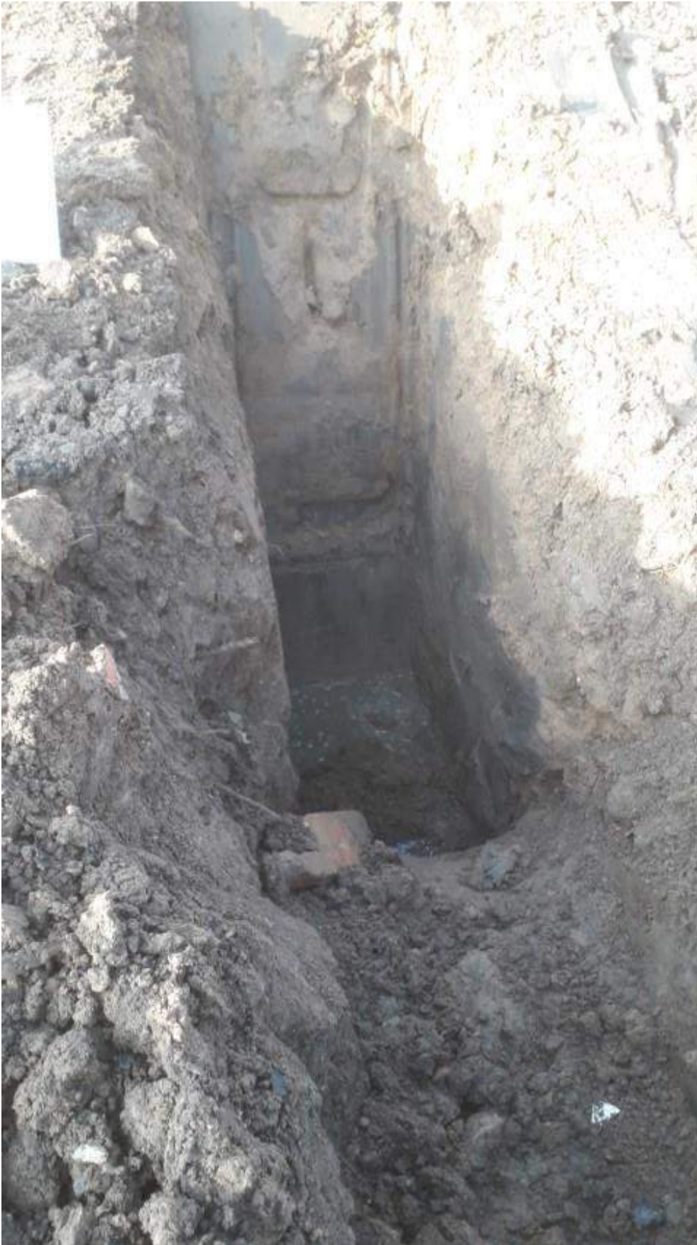
TP101. Bucket scraping on UST brick cradle walls at nearest end of pit.
