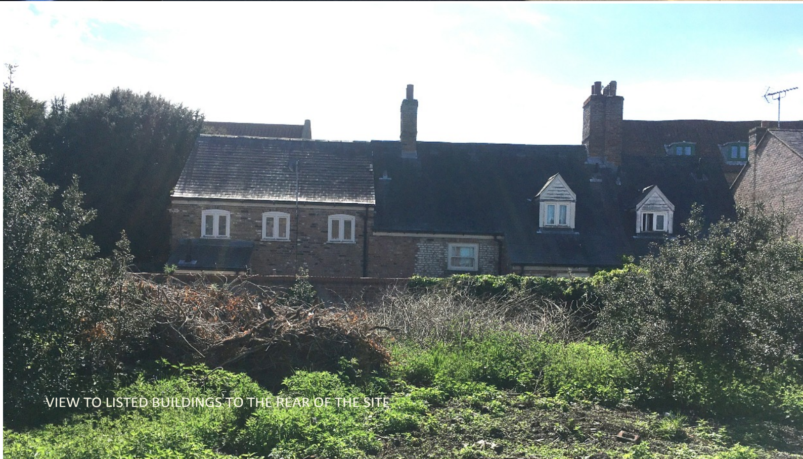
VIEW TO LISTED BUILDINGS TO THE REAR OF THE SITE FROM DOUBLE STREET
