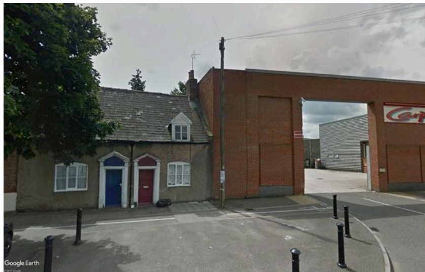
The unfortunate transition between the Grade II listed cottages at Nos.64/65
