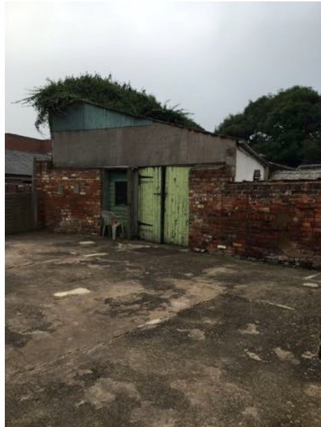
The outbuildings occupying the western arm of the application site
