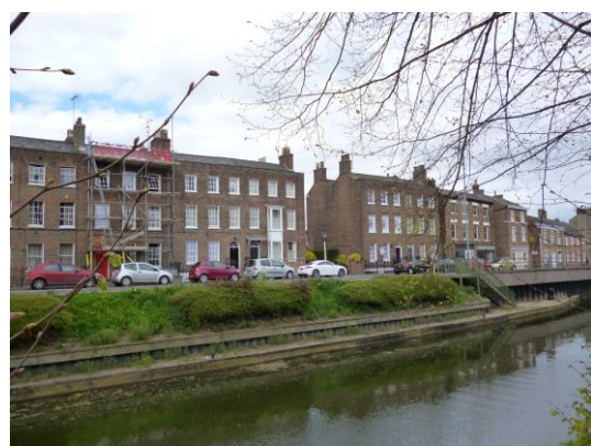
Fig. 02 – Welland Terrace and the streetscene.
