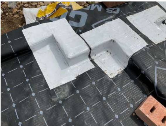
Plot 5. Corner and door threshold details were sealed with SAGM.
