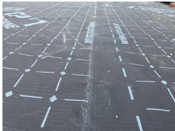
Plot 5. Overview along a hand welded membrane lap joint.
