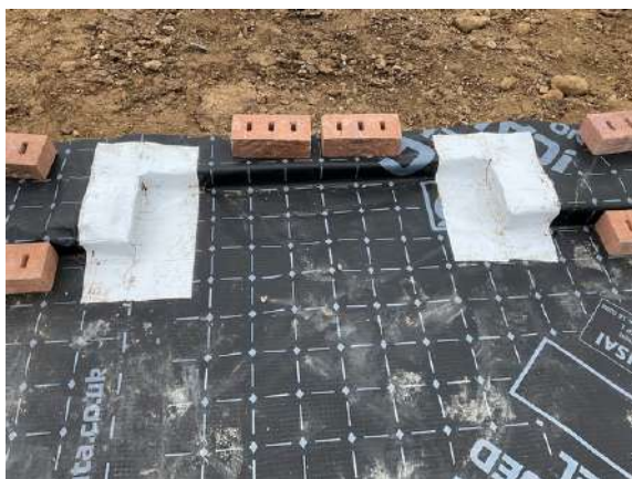
Plot 7. Door thresholds were sealed using SAGM.
