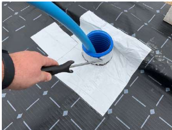
Plot 3. Pick & probe test upon sealed pipe penetration's.
