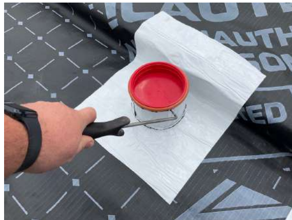
Plot 2. Pick testing upon all sealed pipe entry's.
