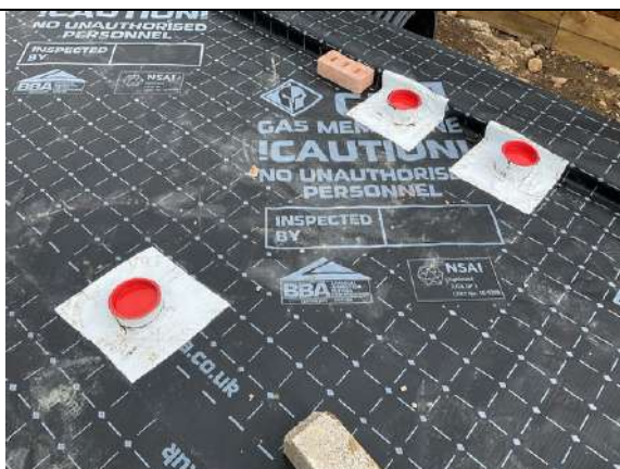
Plot 6. All pipe penetration's were successfully sealed with SAGM.
