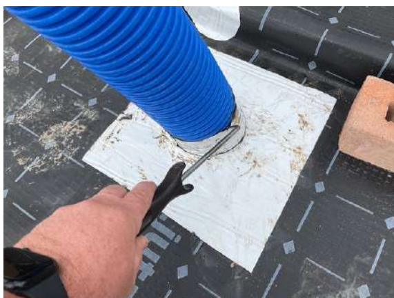
Plot 6. Pick & probe testing to all sealed pipe entry's.
