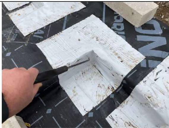
Plot 8. Pick testing to sealed corner details.
