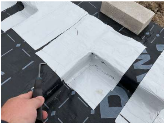
Plot 2. Pick testing to sealed corner details.
