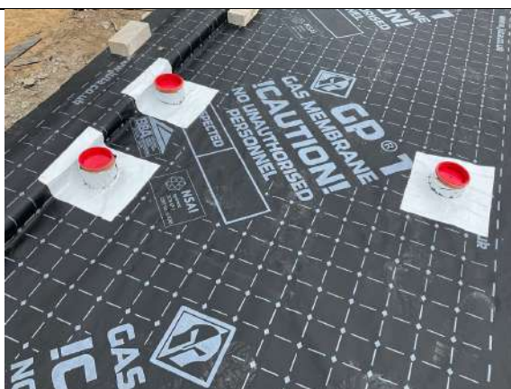
Plot 1. All pipe penetration's were sealed with SAGM.
