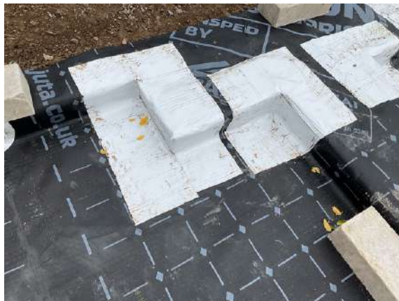
Plot 9. Door threshold and corner details were sealed using SAGM.
