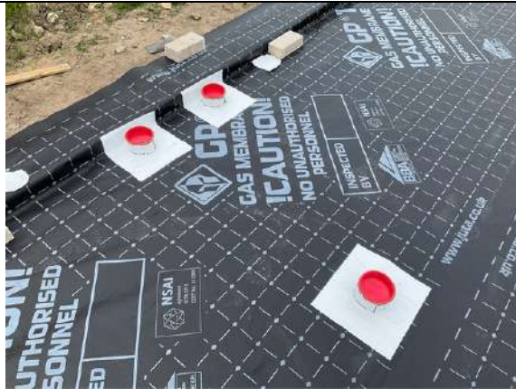
Plot 3. Pipe penetration's successfully sealed using SAGM.
