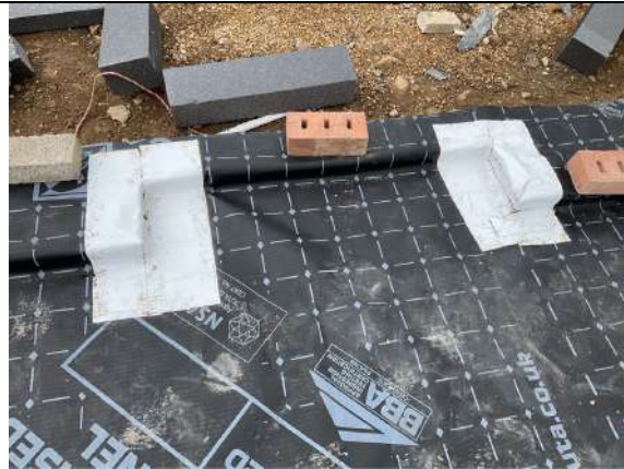
Plot 4. Door threshold details sealed using SAGM.
