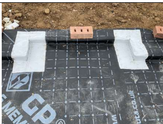
Plot 6. Door threshold details sealed with SAGM.
