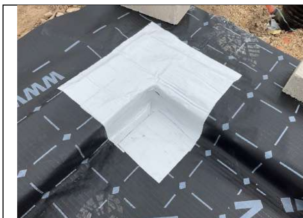
Plot 1. Corner details were sealed using SAGM.
