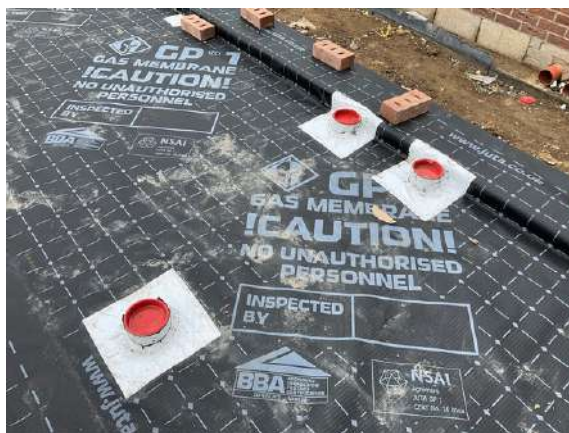
Plot 7. Pipe penetration's sealed using SAGM.
