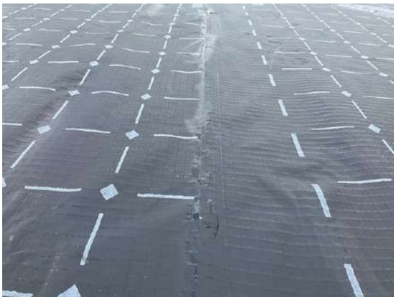
Plot 3. Overview along a hand welded membrane lap joint.
