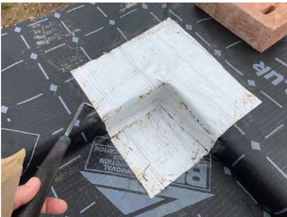
Plot 4. Pick & probe testing to sealed corner details.
