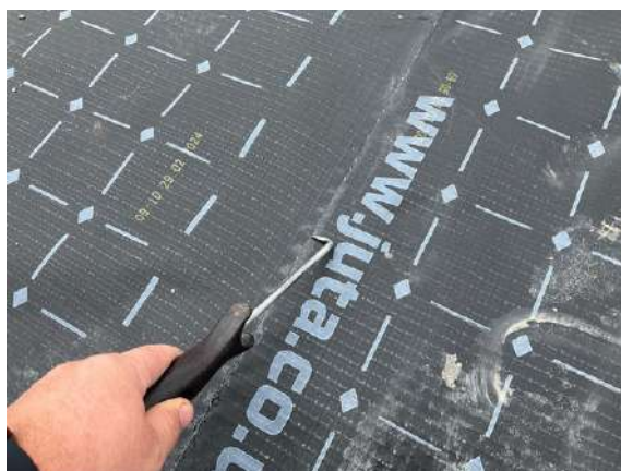
Plot 7. Pick testing along hand welded lap joints.
