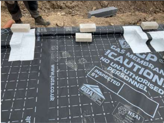
Plot 1. Door threshold details successfully sealed using SAGM.
