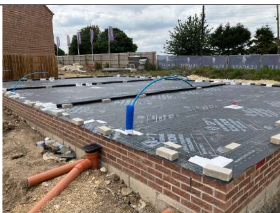
Overview of the full footprint installation to Plots 1-2-3.
