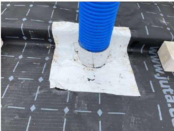
Plot 8. Pipe penetration's were sealed with SAGM.
