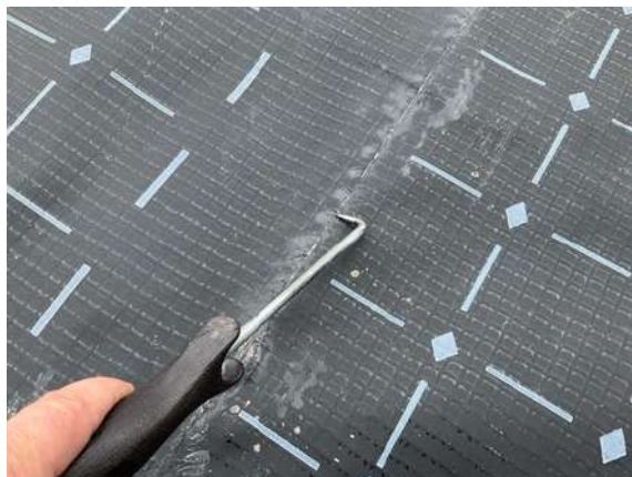
Plot 9. Pick and probe testing along all hand welded lap joints.
