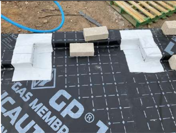
Plot 3. Door threshold details were sealed with SAGM.
