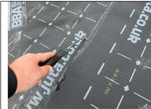
Plot 8. Pick & probe testing along hand welded lap joints.
