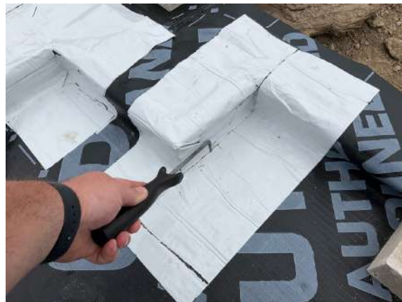
Plot 2. Pick & probe testing to sealed door threshold details.
