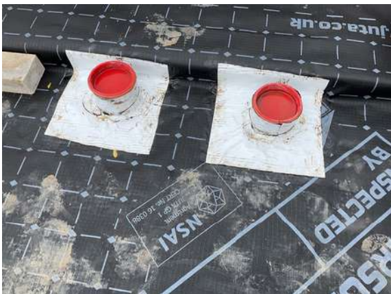
Plot 9. Pipe penetration's were successfully sealed with SAGM.
