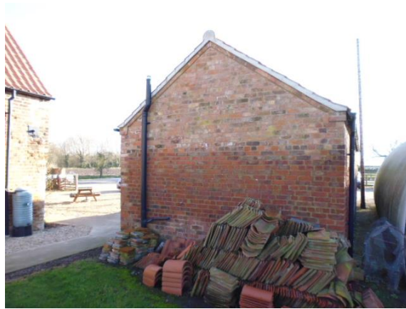
Fig. 04 Gable to which extension is to be added.
