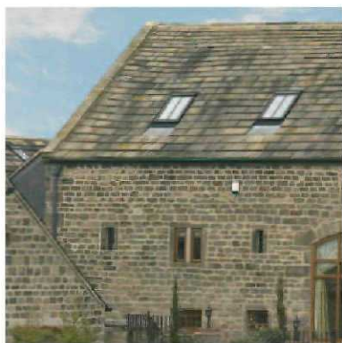
Centre-pivot and top-hung windows.
